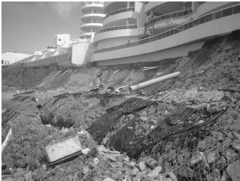
Figure 1.3: Photo taken at Ballito showing the beach erosion (Smith et al., 2007).
