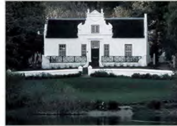
Cape Dutch Architecture (In degrees of wealth): cob walls painted in lime for water proofing - later fire bricks were used
