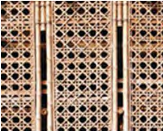
Figure 2.5: DESI centre Screen - The intricate bamboo screen inspired by local techniques but reinforced to use at large scale [Available at: http://www.google.co.za/Heringer/DESI Trainingcenter ]
