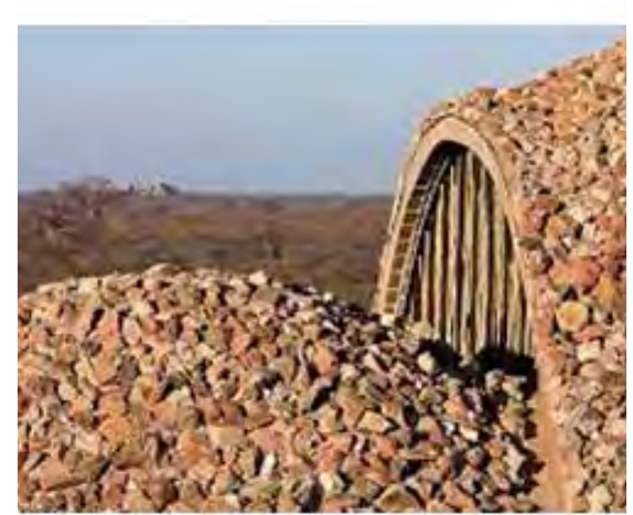
Figure 2.3: Mapungubwe Centre Exterior - Using natural stone from the surrounding hills [Available at: http://www.architectureindevelopment.org ]
