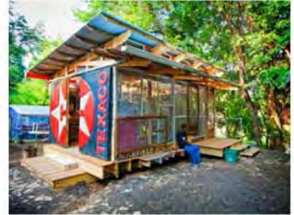
Figure : Burton Street Peace Garden's Learning Pavilion by the Asheville Design Center - Front Elevation
