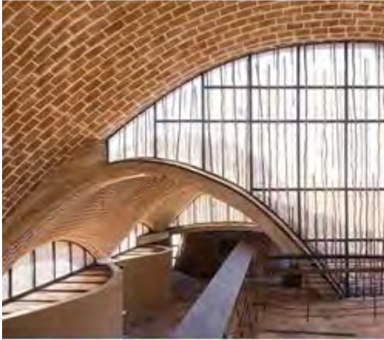
Figure 2.2: Mapungubwe Centre Interior - Using cob bricks and eucalyptus stalks to build the main shell [Available at: http://www.architectureindevelopment.org ]
