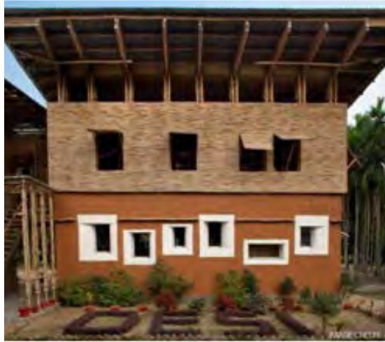
Figure 2.4: DESI centre Elevation - The building's ground floor is constructed mainly from clay with a lighter second floor made from bamboo. (Heringer, 2015) [Available at: http://www.google.co.za/Heringer/DESI Trainingcenter ]
