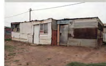
Very poor communities: build out of waste (especially 2nd hand corrugated iron sheets)
