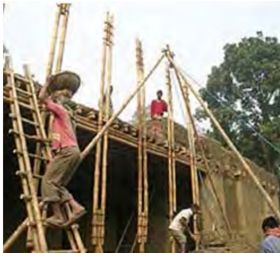
Figure 2.6: Local people building DESI centre [Available at: http://archrecord.construction.com/features/humanitarianDesign/images/0810heringer2.jpg ]
