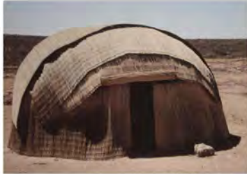
Matjieshuis: Reed mats on a timber structure moving around for new grazing fields (Khoi-San & temporary settlement for Dutch settlers)
