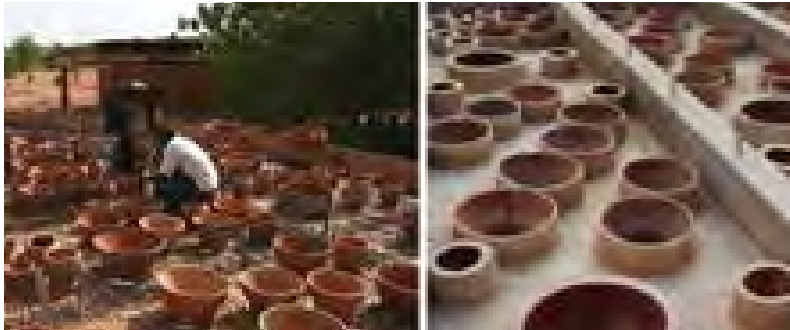
Figure : Francis Kere's Library Roof being prepared for setting [Available at: https://www.google.co.za/search?q=francis+kere+library+clay+roof ]
