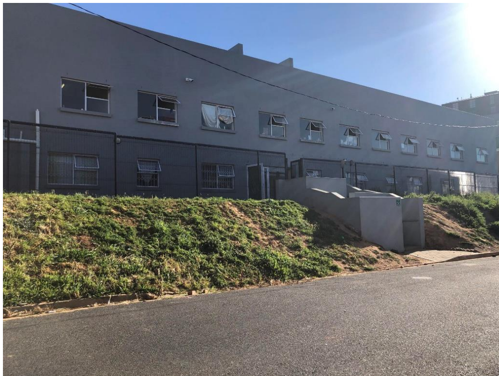
Figure 1.1: The case under study: The Pickwick Transitional Housing Project (Source: GroundUp, accessed September 2023)
