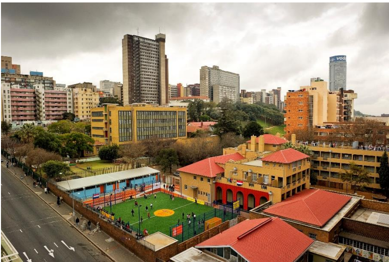
Figure 4.16: BG Alexander facility (Source: Google image, Rooftops Canada, accessed September 2023)
