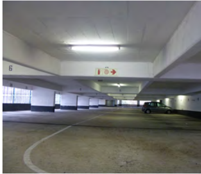
Figure 57: Parking garage floors 2-7
