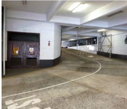
Figure 56: Vehicle ramps floors LG -1
