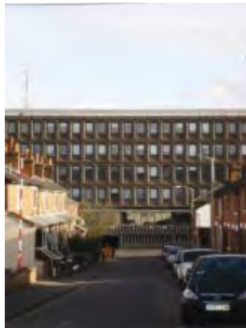
Figure 20: The original 1960's façade of the Elizabeth II Court
