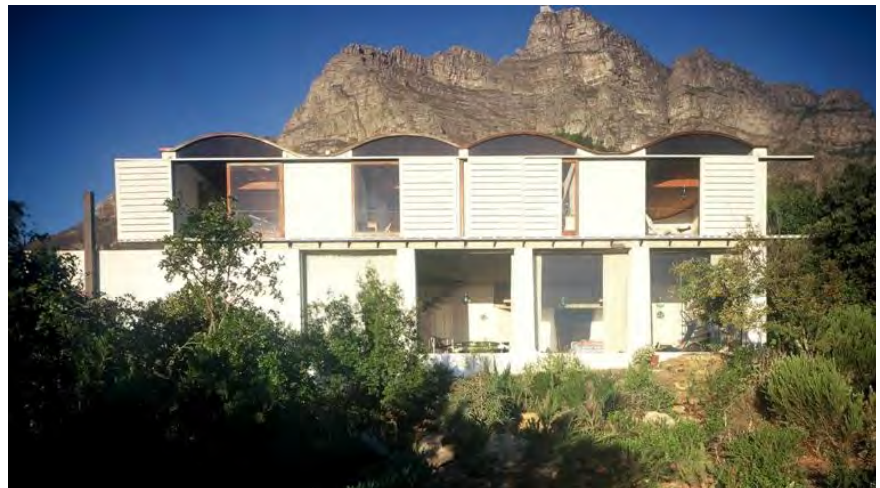
Figure 12: East facing windows protected by adjustable sliding screens in die Es
