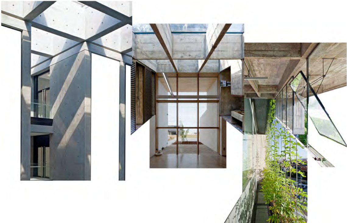
Figure 90: Collage of exposed concrete surfaces, concrete frame roof structure and openable windows creating a naturally lit and ventilated interior space
