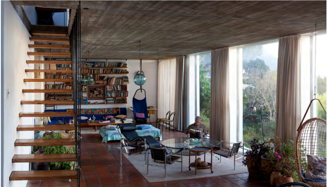
Figure 19: Thick external load bearing brick walls along with the tiled floor and a thick first floor concrete slab create a heat sink. Daylighting and natural ventilation enhance the lovely open plan environment
