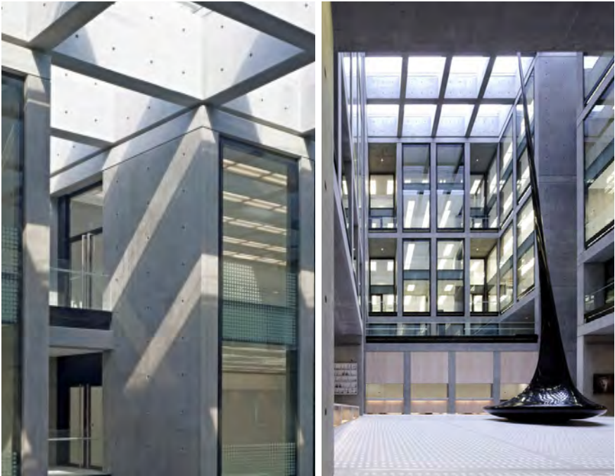
Figure 25 & 26: The thermal mass and control of internal environment has contributed to the 'Excellent' BREEAM (assessment method for sustainable buildings) rating of the Angel Centre
