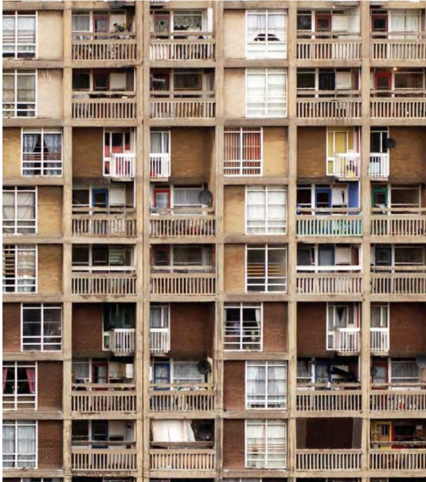
Figure 35: Park Hill in Sheffield was a council housing estate built between 1958-1961 and designed by architects Ivor Smith and Jack Lynn. The building is made up of a series of interconnected blocks constructed using concrete frames
