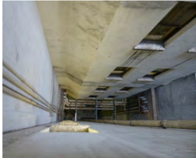
Figure 58: The main light well is halved in two due to the later inserted goods lift
