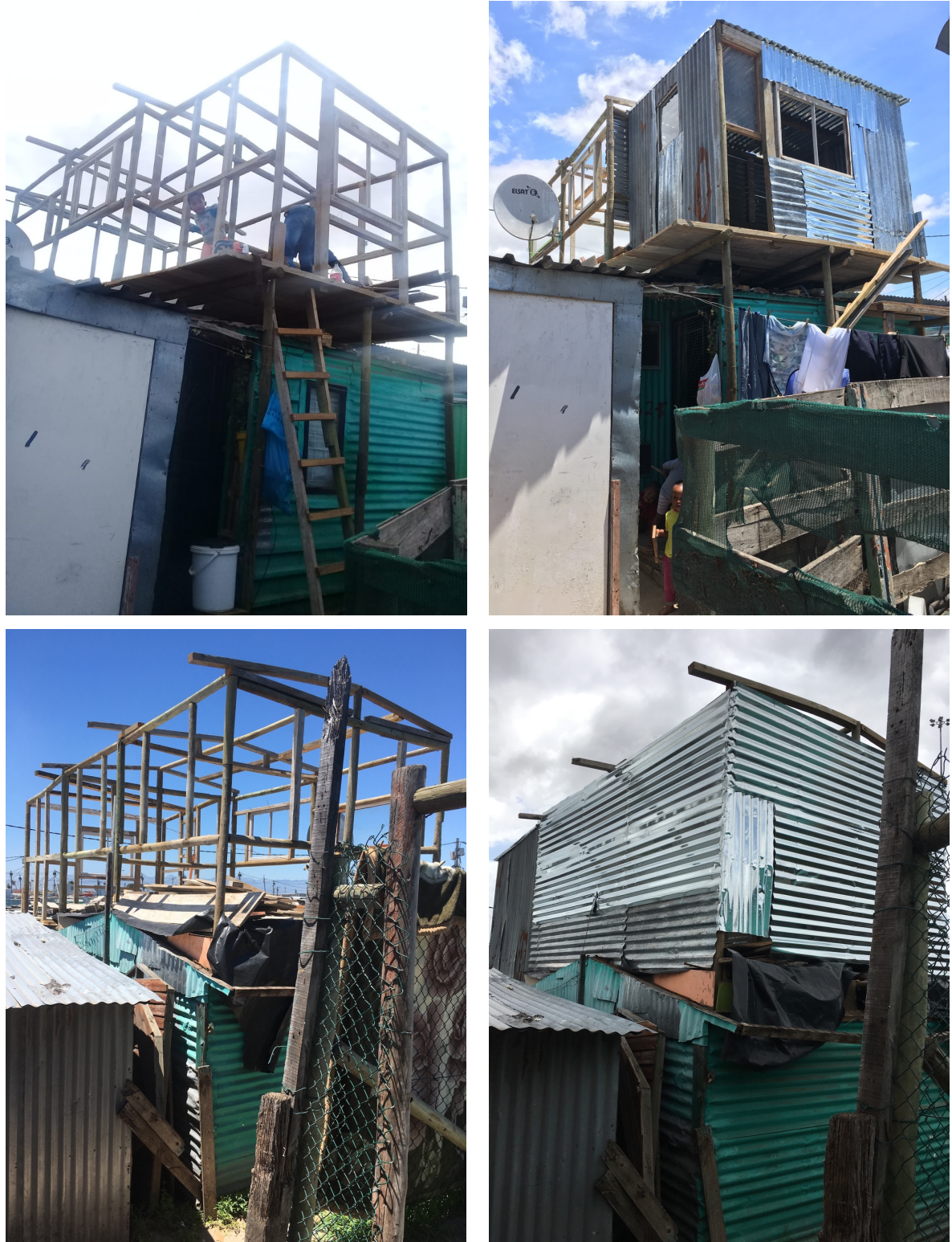
Plate 3.9: Under construction double storey of PO's shack in Kosovo
