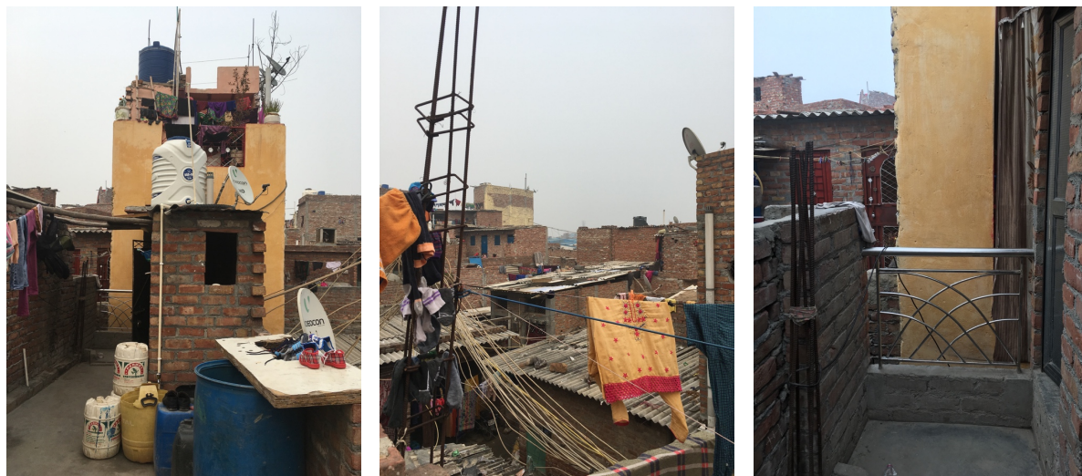
Plate 4.4: ID’s current terrace in Gayatri Colony with toilet and potential for adding more floors
