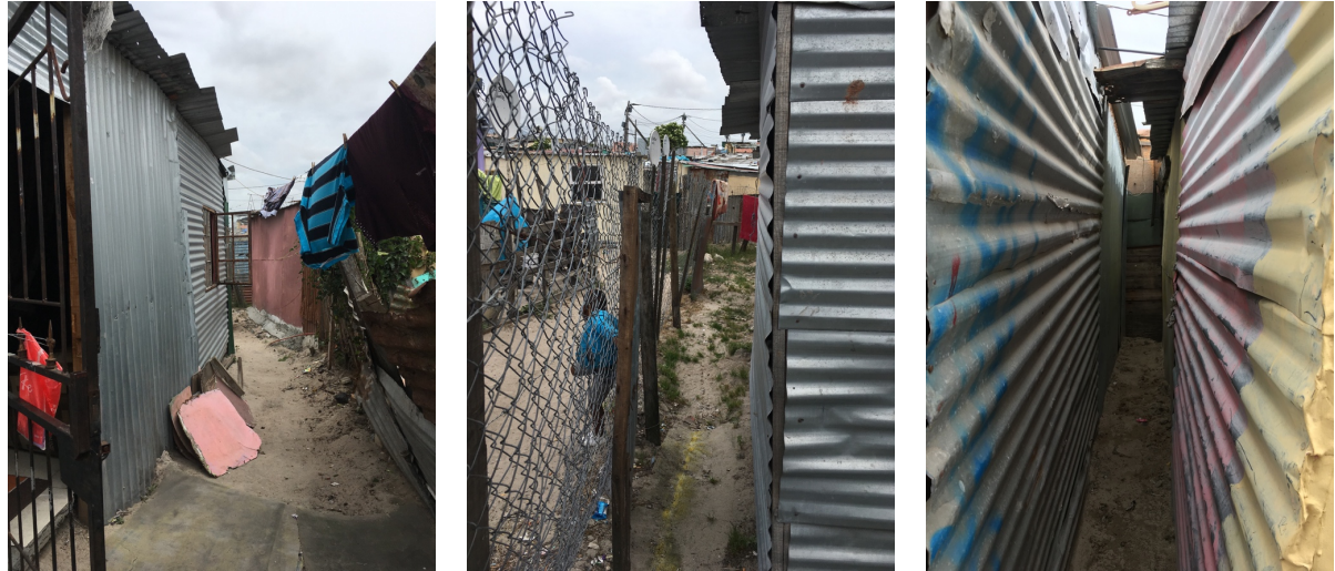
Plate 3.3: Keeping distance between shacks to Prevent spreading of fire in Kosovo
