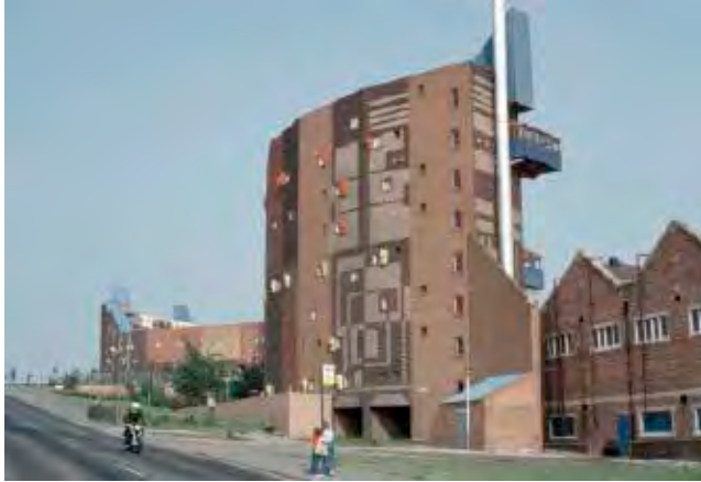
Figure 8: The Byker 'wall' creates a sense of a neighbourhood enclave. Small windows face the busy road to reduce noise. (Anon, 2010)
