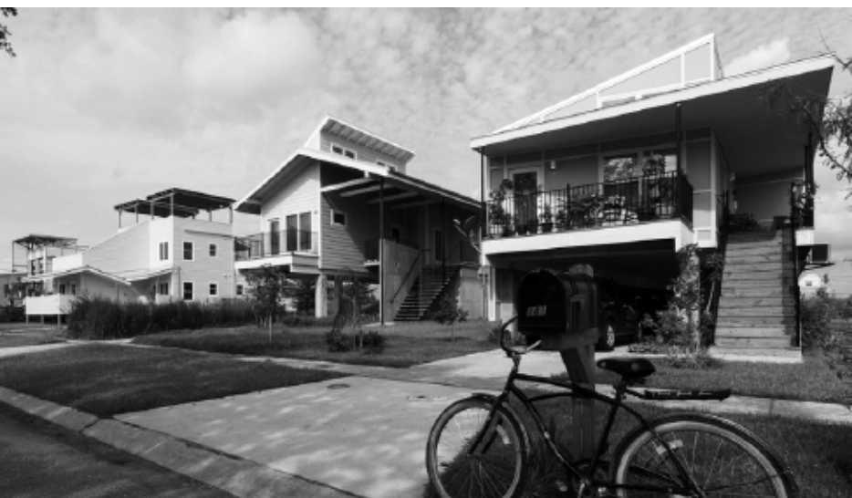
Figure 50: (Left) The neighbourhood of 'Make it Right' houses. The houses in the foreground are raised high enough to create parking space under the building. (Right) The 'Make it Right' house by Frank Gehry. (Make it Right, 2012)
