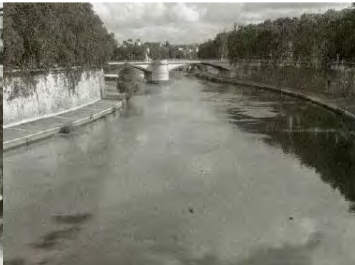
Figure 49: (After) The Tiber River in Rome after the river was canalised with tall walls. Buildings were demolished to create this canal. (Nonderson and Seavitt, 2011: 43)
