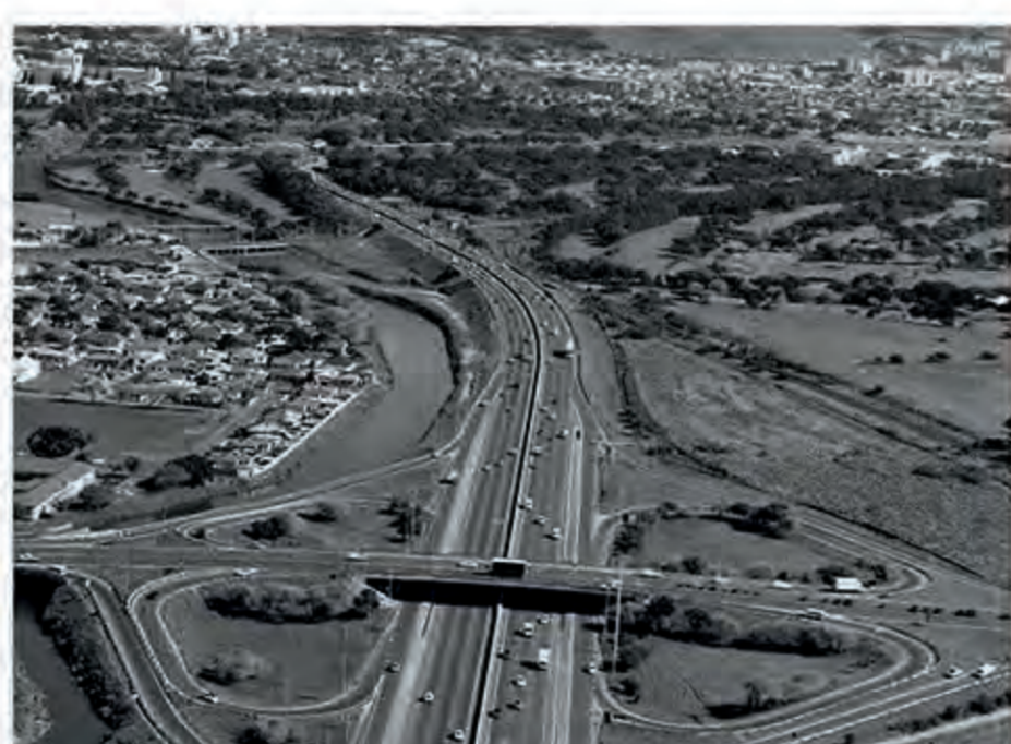
INADEQUATE CONNECTION TO NEIGHBOURING SUBURBS
