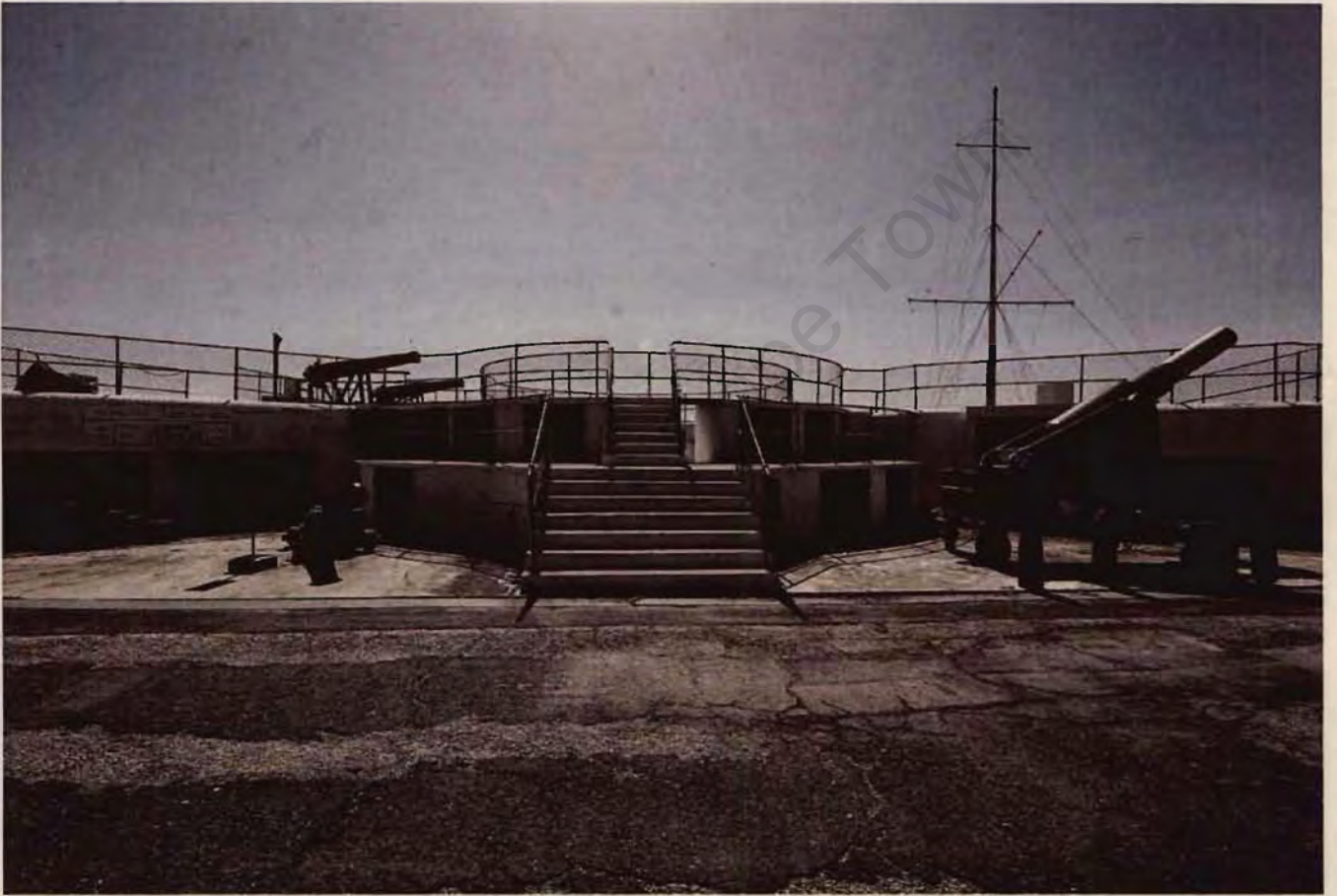
Figure 13. The empty gun site with all its supporting services and protective concrete work as well as a collection of older cannons moved here when the site was opened to the public.
