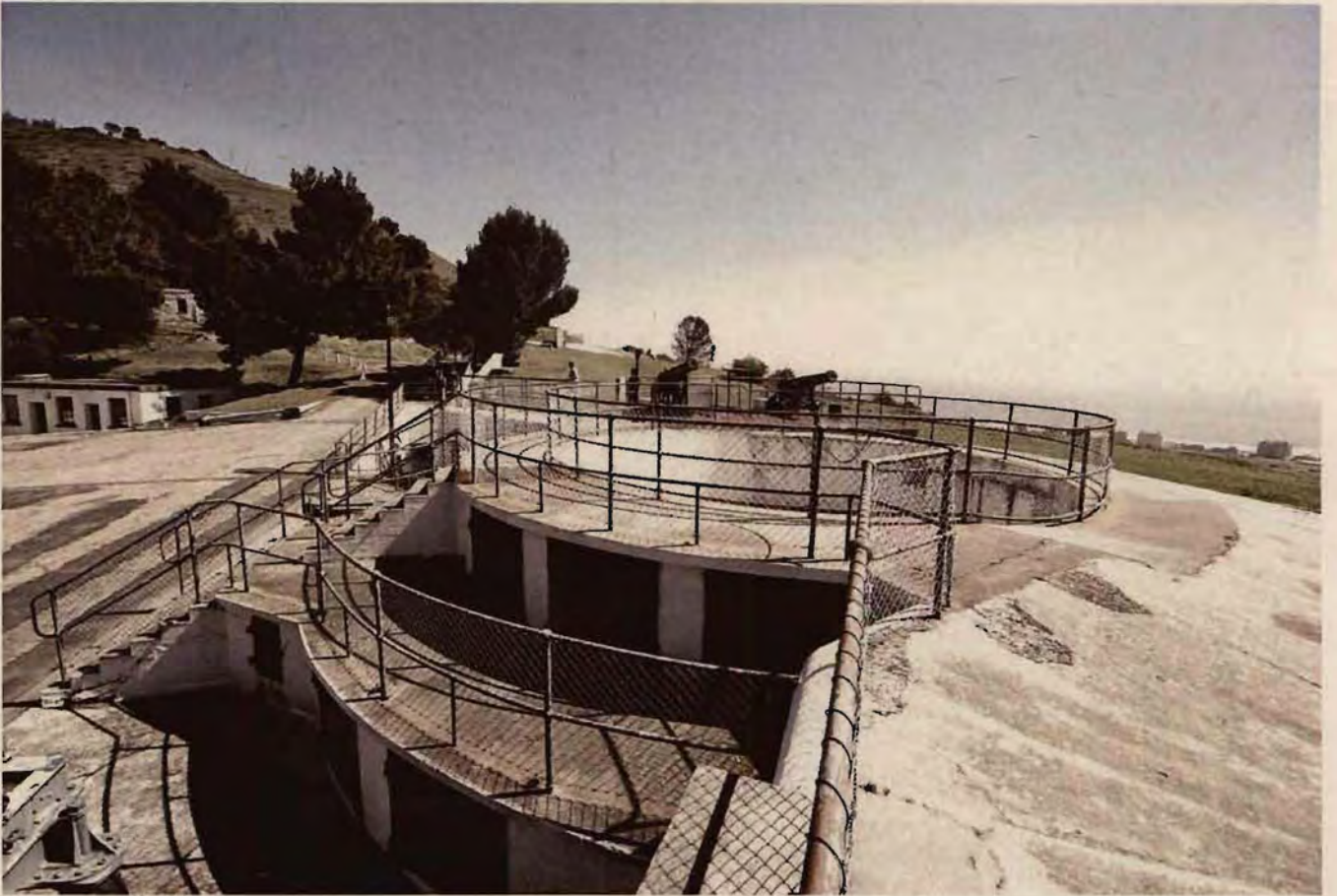
Figure 11. The empty gun site with all its supporting services and protective concrete work.
