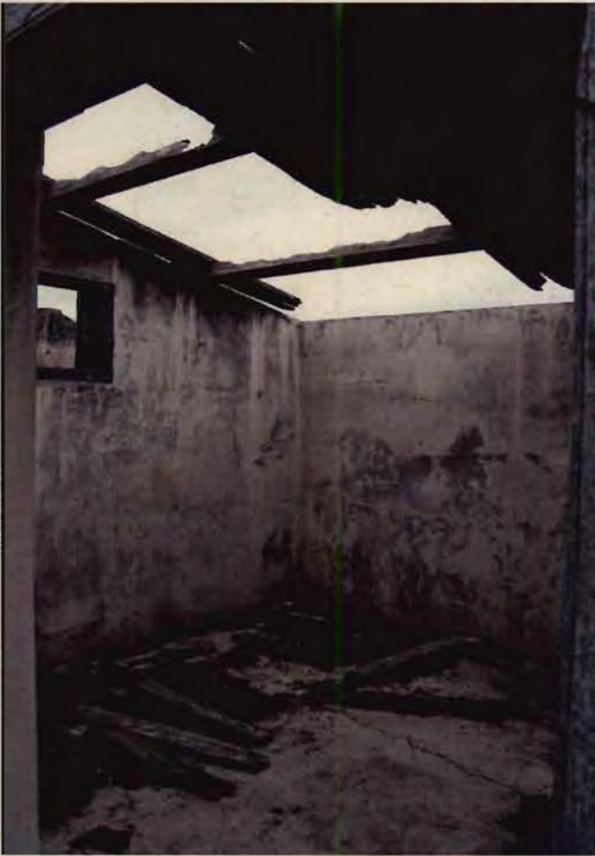
Figure 35. Burnt out radio room.
