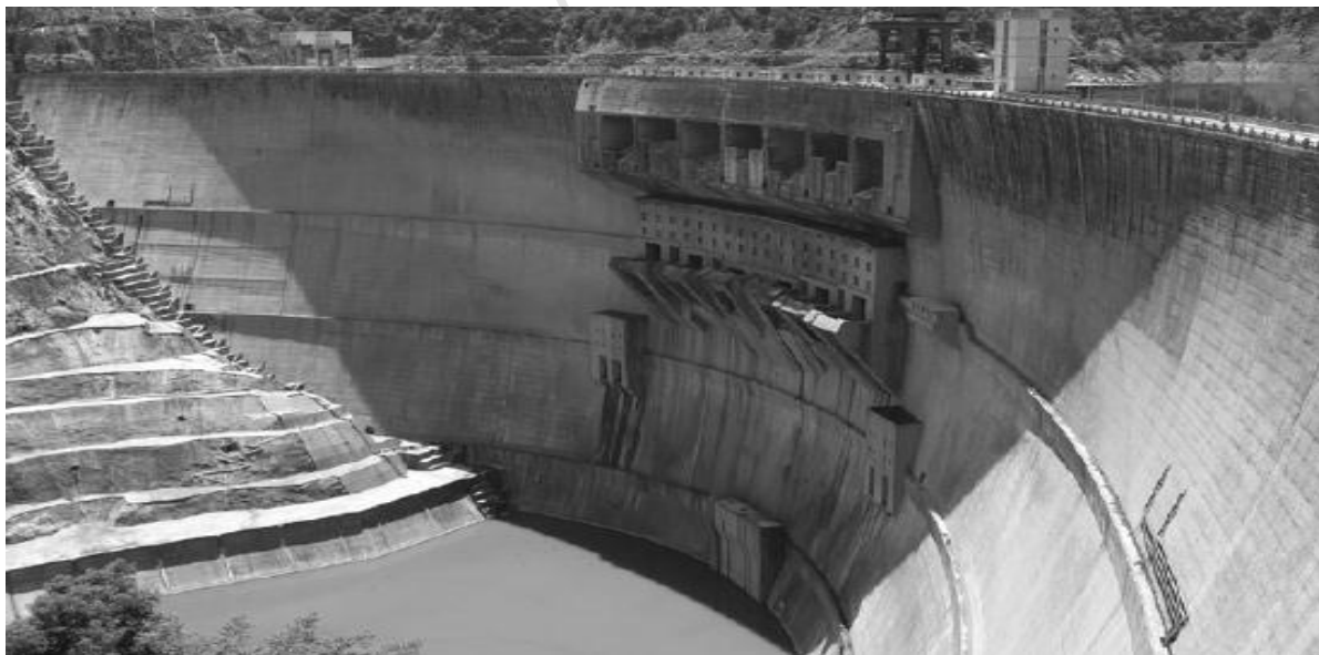
Figure 2.5: Illustration of direct solar radiation and shading effects on an arch dam in China (14h00, 02 August 2006).
