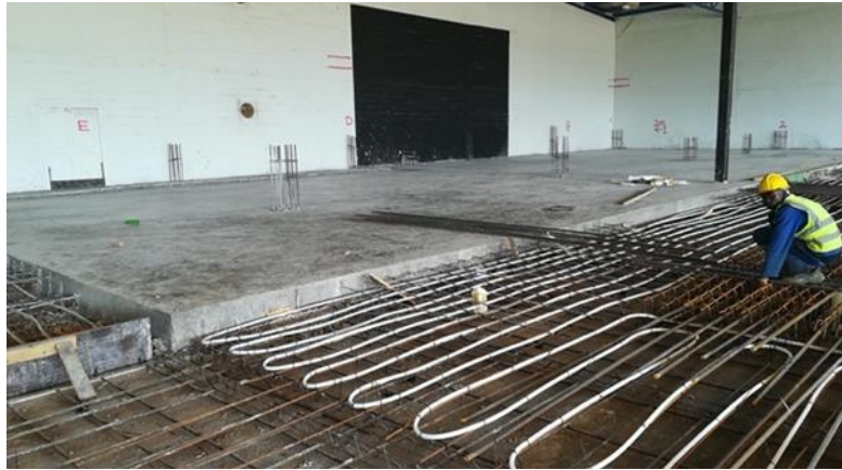
Figure 5-4: Pipe Installation and Poured Cement
