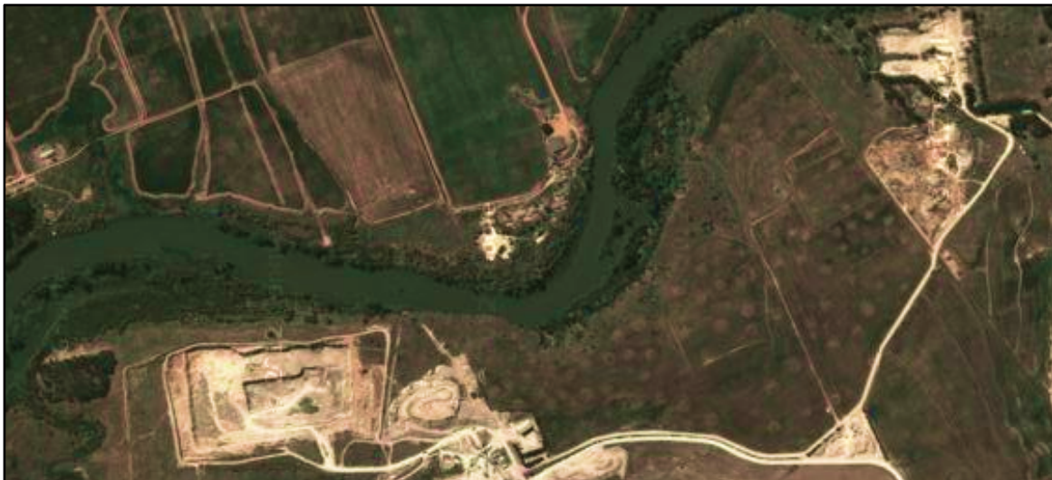
Figure 5.5 – Quarry located on the western bank of the Berg River, near Saron (Image courtesy of Google Earth, 2013)
