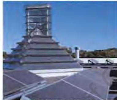
Image taken from the roof showing the solar panels and the 'lanterns'.
