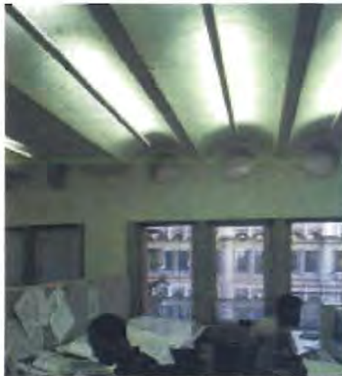
Heat which the lighting generates is directly absorbed into the vaults. Vaults extrude through the envelope to create balconies.
