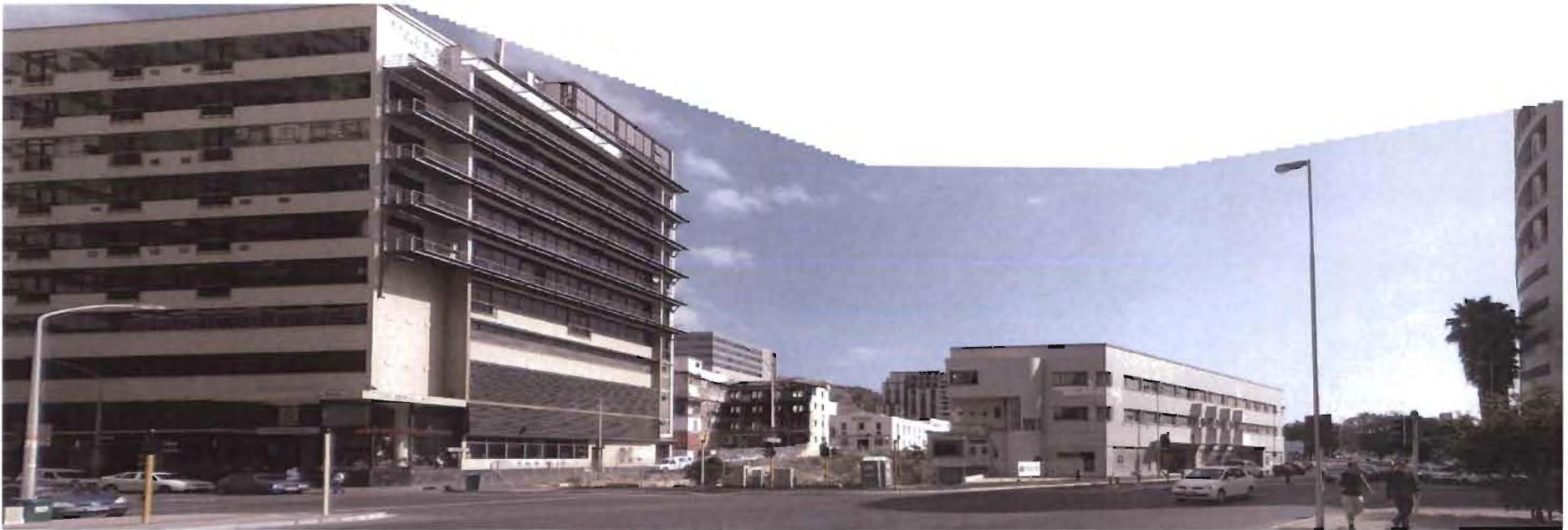
View from South of Site
