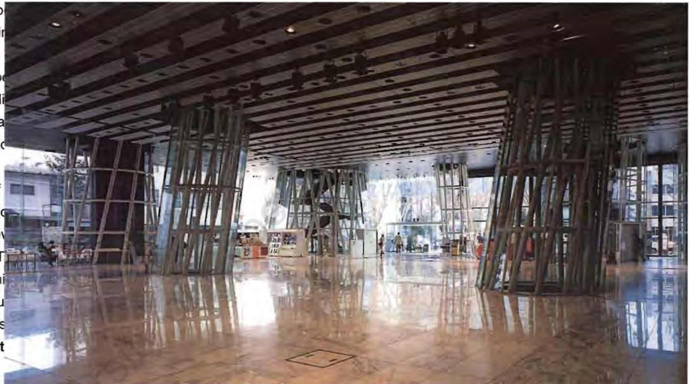
Seemingly irregular spacing of tubes inhabited by different functions. The different structural patterns can be seen due to the tubes location, size and angle of inclination
