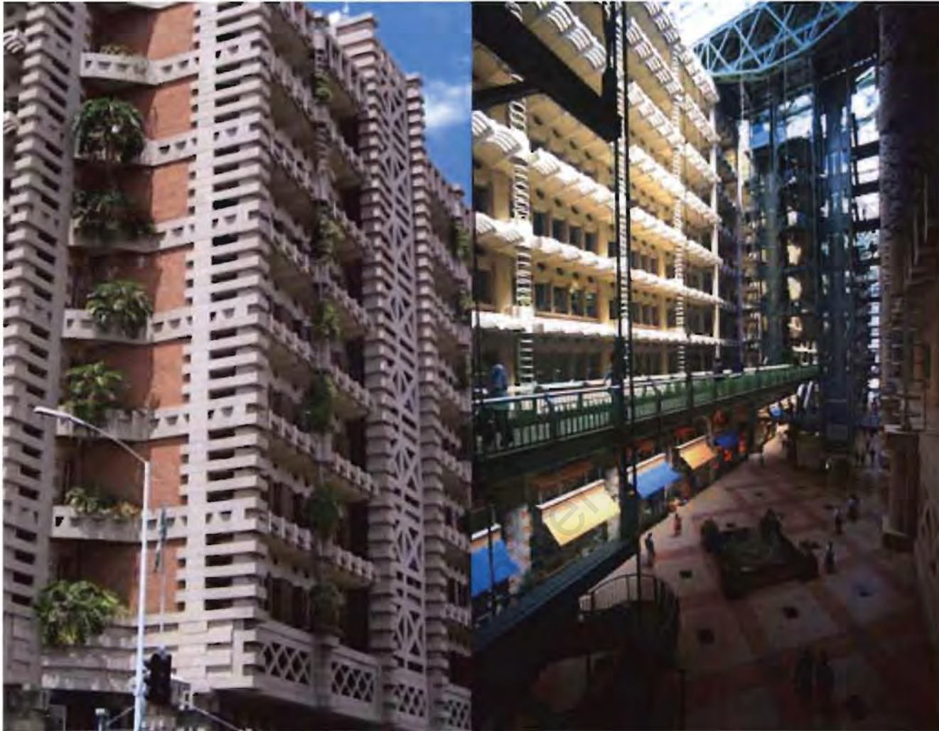
Eastgate building external 'heavy' expression is responding to nature, Eastgate interior atrium creates a public space and accommodates appropriate resources and attending to cultural language. culation - a mix of delicately detailed lattice girders make up the sky light roof.
