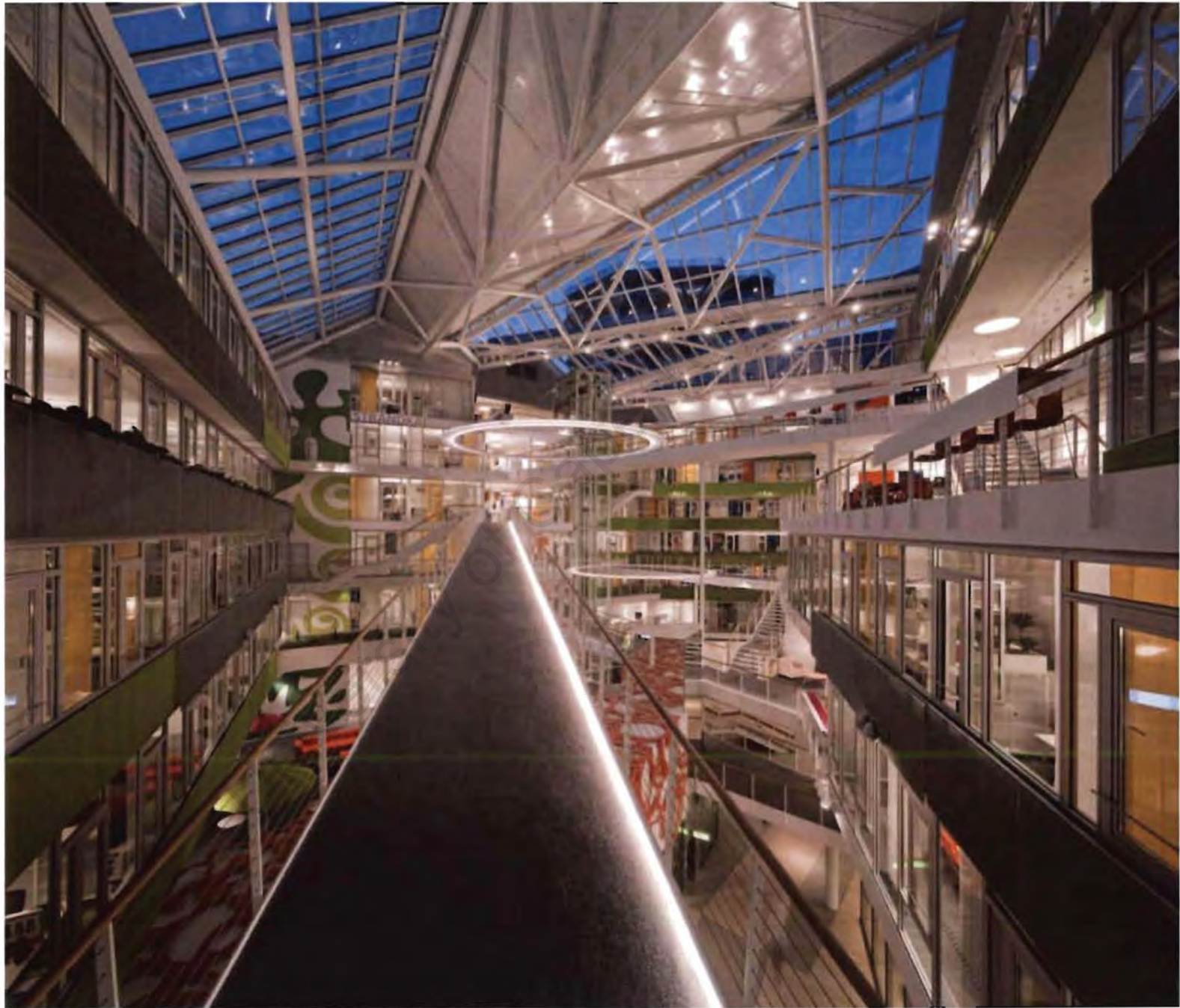
The saw tooth nature of the roof structure is such that it creates a sculptural folding feature. The roof structure and ramps expresses the idea of connectivity and networking between people.
