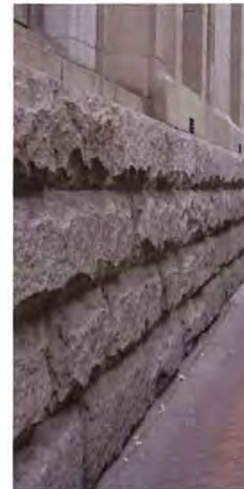
Figure 53. Textured with deep reliefs means that it will diffuse sound, and cast shadows
