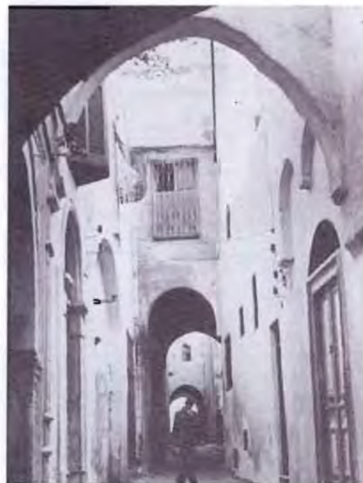
Figure 106. A cul-de-sac street showing a sabat , or a room bridging the street
