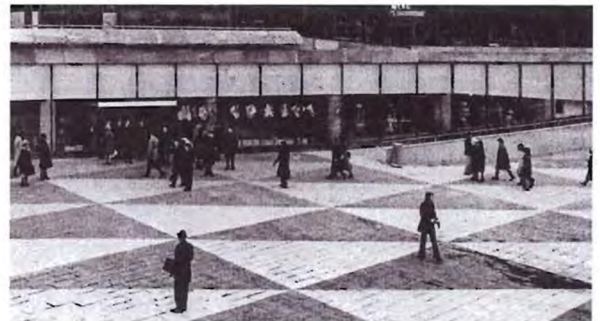
Figure 60. This ornamental triangular paving pattern visually subdivides the large open space.
