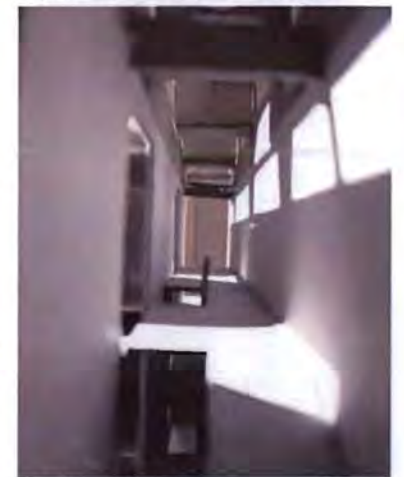
Service wall lighting
