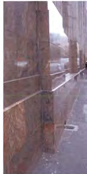
Figure 52. Smooth granite wall, Darling Street, Cape Town, reflects sound and light
