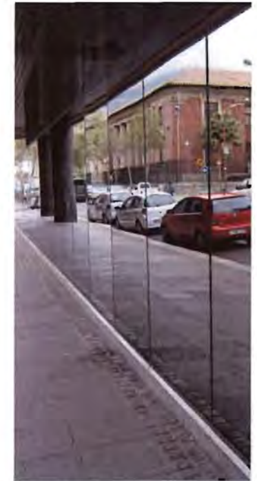
Figure 54. Shear glass wall, highly sound reflectant at high frequencies, Caledon Street
