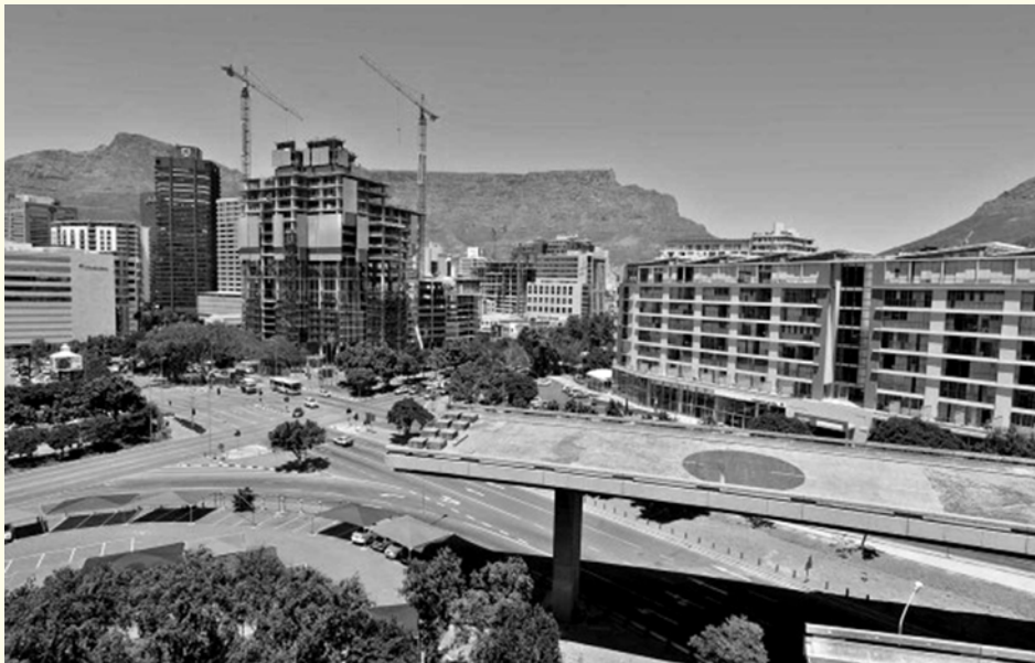
The unfinished overpass.
