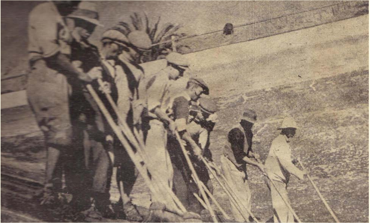
Cleaning of Molteno Reservoir, Oranjezicht, Cape Town, Cape Times 1927.
