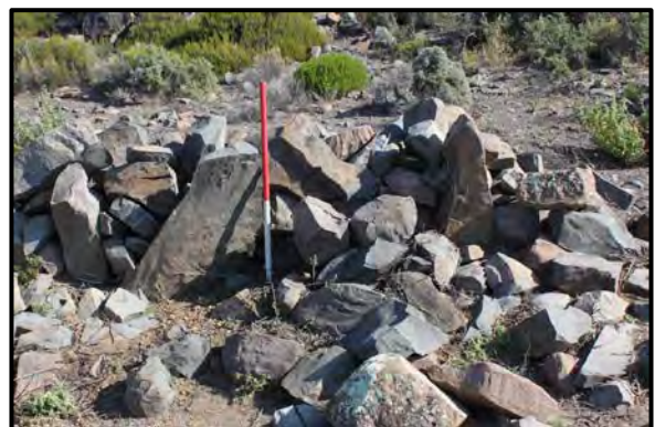
Figure 5.5.4. Exterior section of kraal 01 at WG01. Not in a very good condition but it possible to see the similarities with the Scholtzenhof wall in Fig. 5.5.3.
