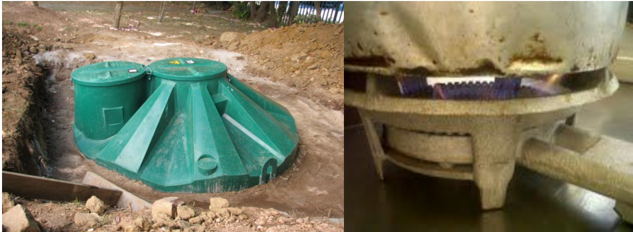
Figure 6.1: The Leo Marquard Hall Biogas Digester
