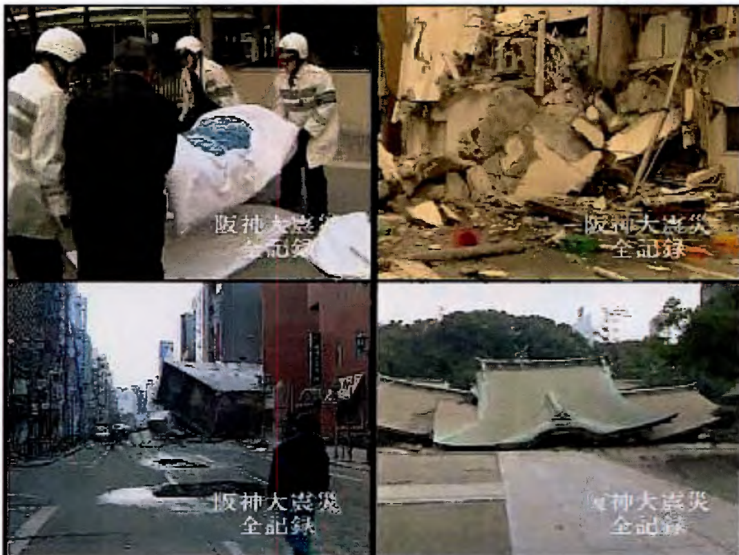
Figure 1.3.: The devastation caused by the Great Hanshin-Awaji Earthquake [6].
