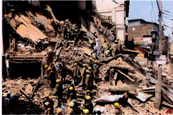
Figure 1.1.: The collapsed Kashmir building in Srinagar, India on the 21 st August 2009 [4].
