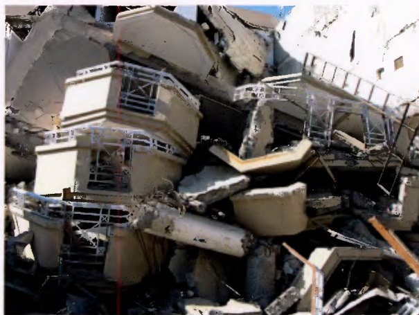
Figure 1.2.: Destruction in the Canterbury region owing to the 2011 Christchurch earthquake [5].
