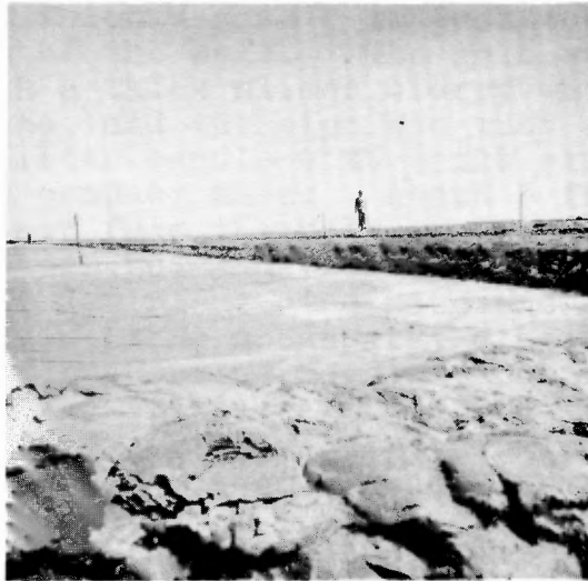
(b) Top of buttress wall showing tops of piezometers.
