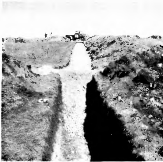
Graded material in drainage trench.
