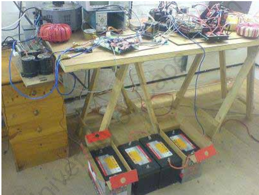
Fig 4.16: The 4 12V battery cells used to test a 24V, 36V and 48V configuration
