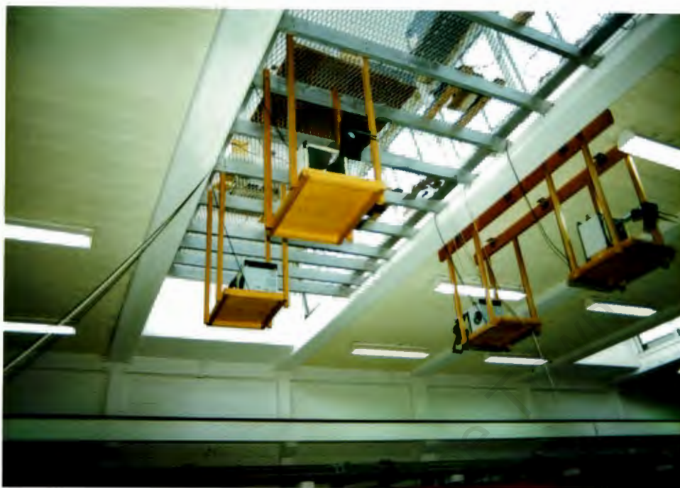
Plate 5.12 Overhead projectors mounted on the ceiling.
