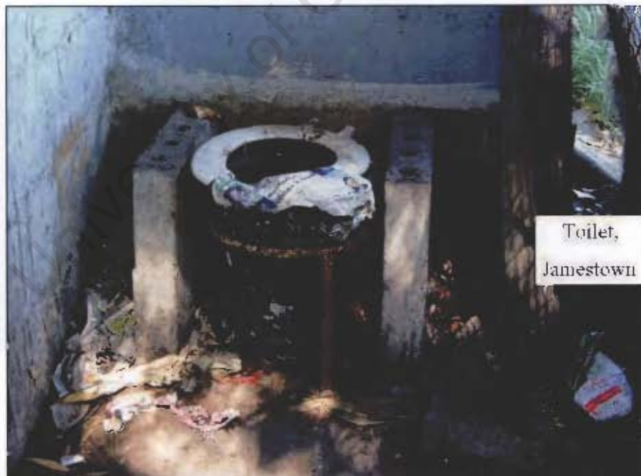
Figure 20: A Bucket Toilet
