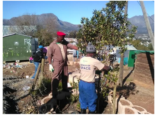
Figure 5.6 The community of Langrug planting trees in catchment pits connected to greywater disposal pits, courtesy: GOS, 2016
