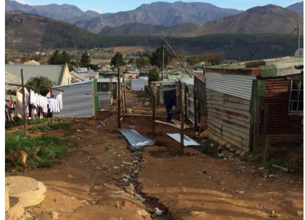
Figure 5.2 A view of an open stormwater channel in Langrug, courtesy: GOS, 2015
