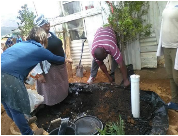
Figure 5.5 The community of Langrug planting trees in catchment pits connected to greywater disposal pits, courtesy: GOS, 2016
