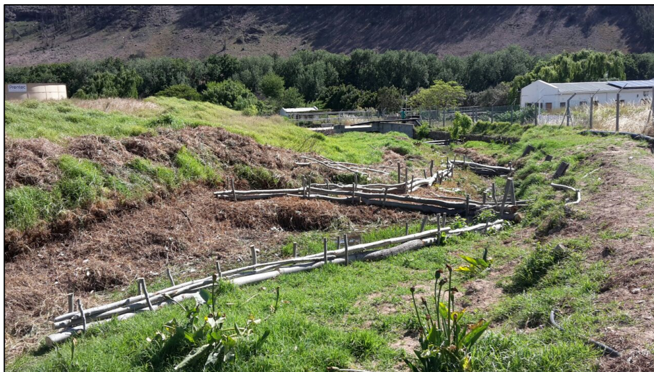
Figure 12: The construction of the rehabilitated section of the Stiebeuel River.
