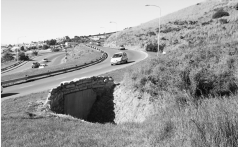
image of the culvert on site
