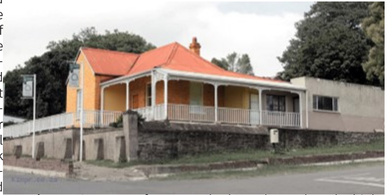
Figure 16: Image of a vernacular home located on the highlighted red intersection on fig.11( https://kznpr.co.za/richmond/nggallery )
