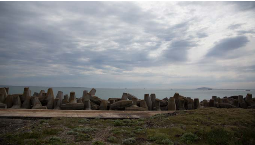
Fig. 19. Coastal armour along the northern face of the wall.
