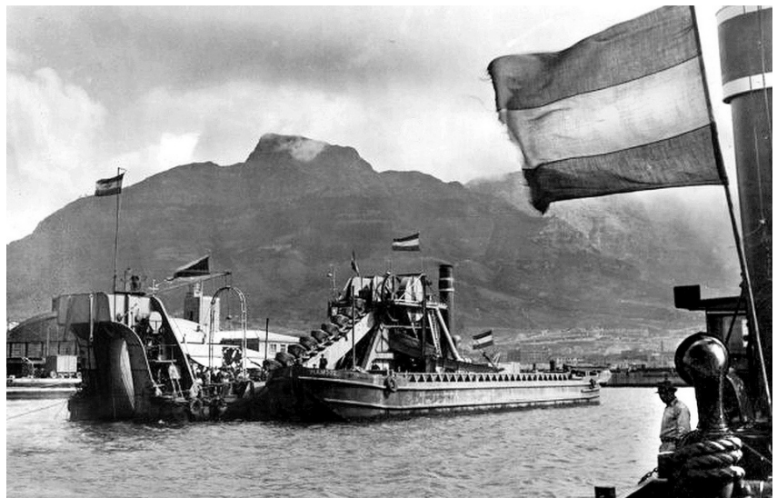
Fig. 10. Dredging vessels constructing the Duncan Docks in Cape Town, 1939.
