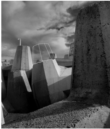
Fig. 33. The Dolos form an unusual terrain along the northern face of the wall.
