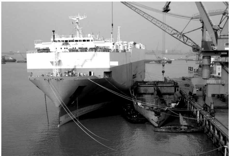
Fig. 45. Quayside breaking taking place in Shanghai, China.
