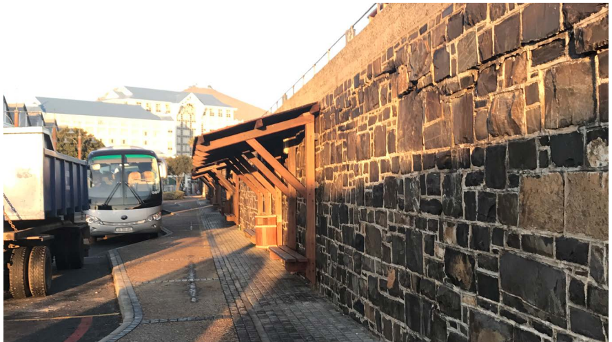
Fig. 22. Peculiar clip-on timber structure as a shelter near the bus stop.
