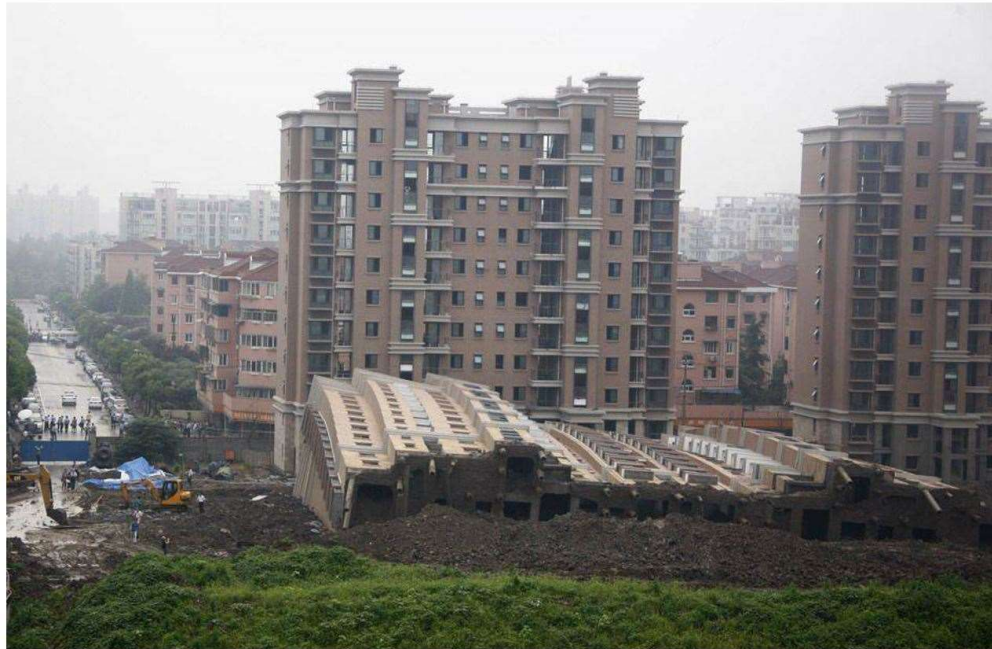
Figure 2-5: Lotus apartment, Block 7, collapse (Chai et al. , 2014).
