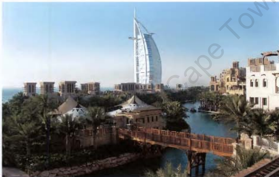
FIGURE 1.2: One view of the extravagant Madinat Jumeirah resort, with the Burj-Al Arab in the background [4]
