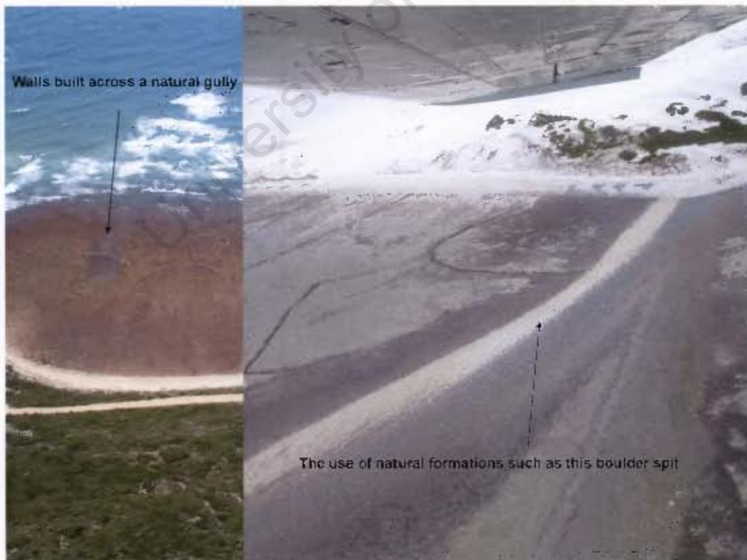
Figure 1.4 Photographs showing the use of natural features in the construction of vwyers.
