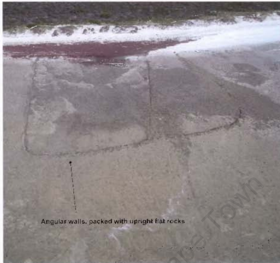
Figure 1.3. Photograph of a vwyer set in the OTB stretch of coastline showing the fully constructed walls on a sandy/pebble intertidal zone.
