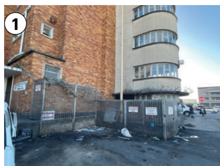
Figure 25 : Areas hidden from public view tend to attract illicit activities and suffer from inadequate sanitation Source: Author (2023)
