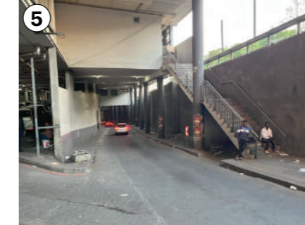
Figure 29: Access point to the subterranean taxi rank. Source: Author (2023)
