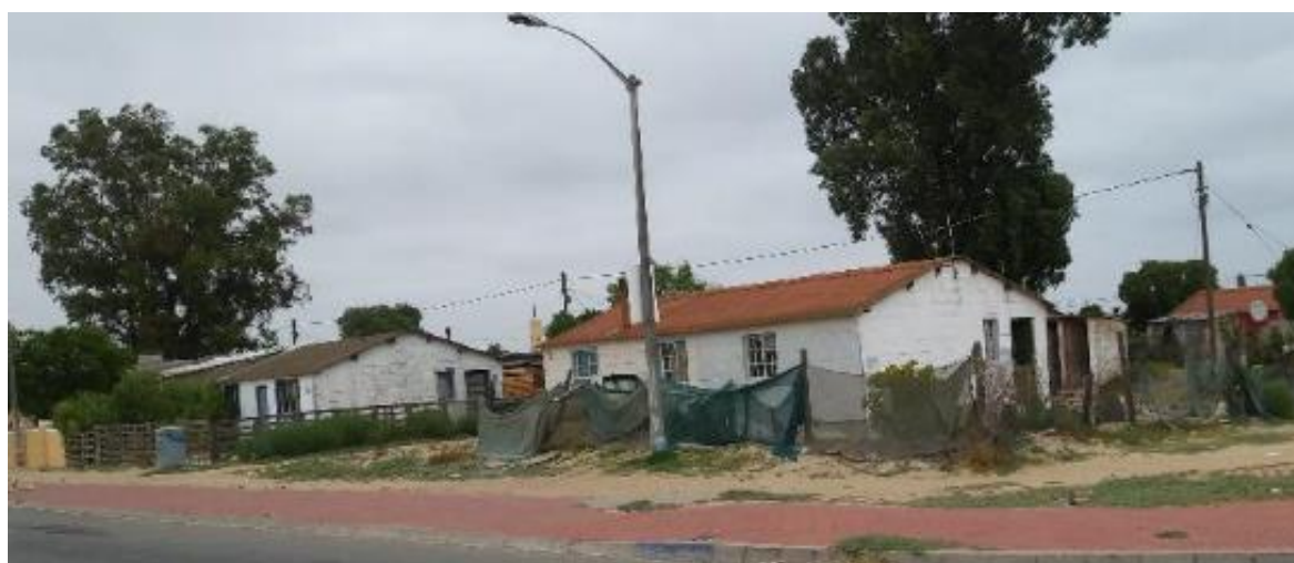
Figure 23: The oldest houses in Noordhoek in the sub-area known as 'Oublok'. (Source: Author's own)
