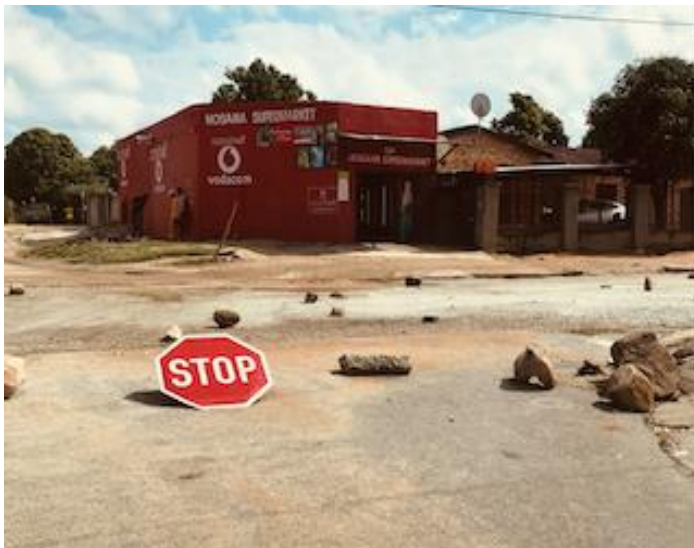
Figure 5: Damage to public roads and infrastructure is a common consequence of protests and can take months, even years, to be repaired. Source: Own photo
