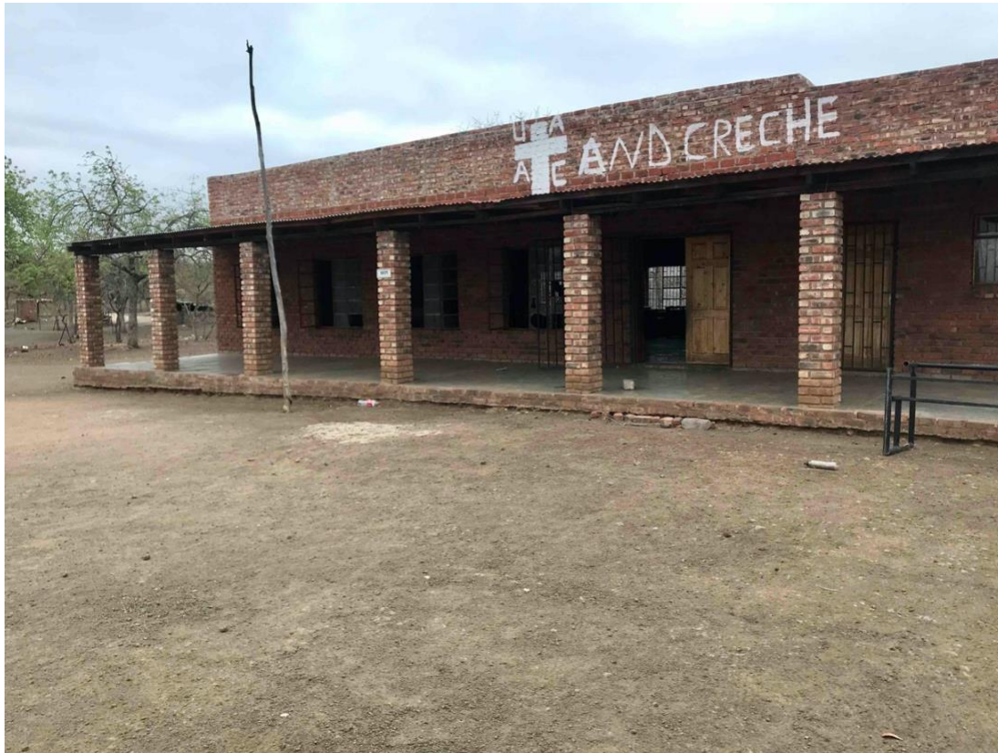
Figure 37: Community hall, village on the northern outskirts of KNP. The building houses community-meetings between the park and people from the village. Source: Own photo.
