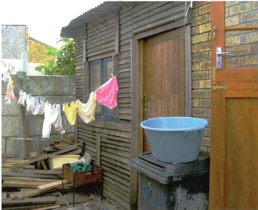
Photograph 6: Backyard Wendy house with no bathroom or toilet
