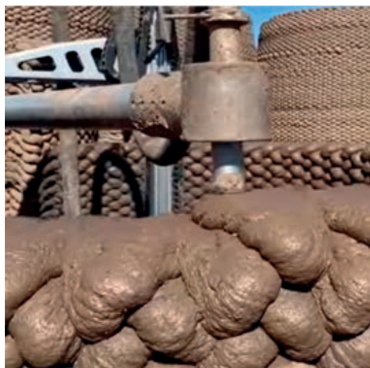
The beading technique used by Emerging Objects in their hut project in Mexico where they exclusively print with the local mud.
