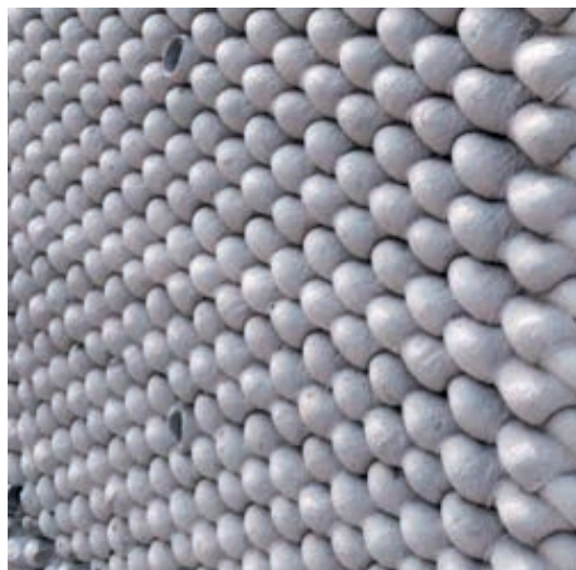
The 'beading' technique used by WinSun to prevent the separate printed layers from sliding off each other when under compression.
