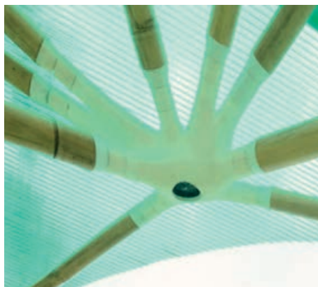
FIG 47 Structurally optimized beams printed using the minimum material required.
