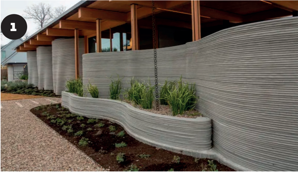
FIG 67 'House Zero' printed by ICON
