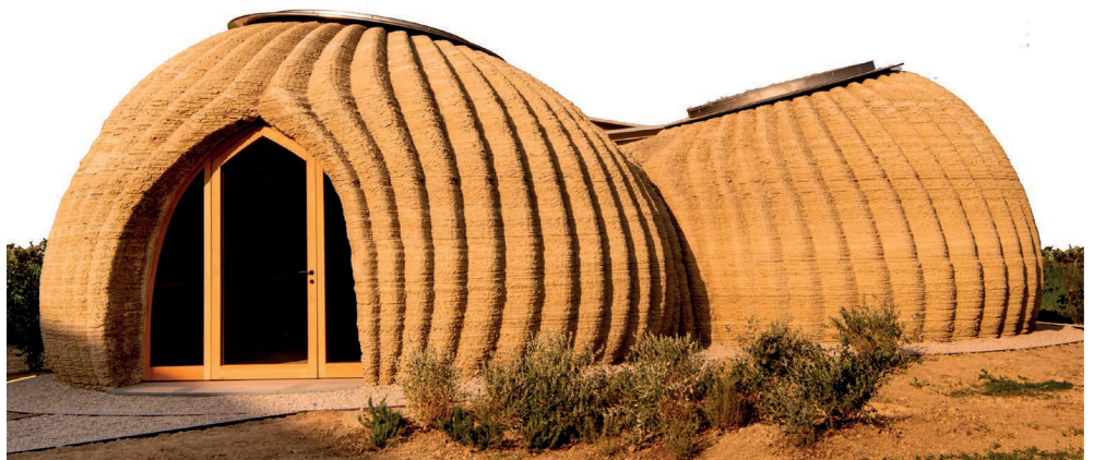
FIG 17 The first ever house printed with earth by WASP architects demonstrates how the architectural language can be a direct product of the construction methods used.
