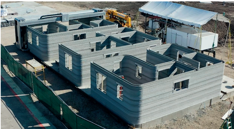
ICON's 3D printed homes in Texas, USA, are examples of the typical load-bearing wall typology 3D printer constructors opt for.
