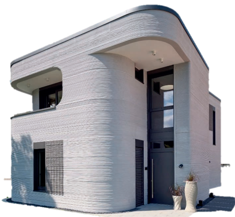
FIG 16 The first 3D printed house in Germany in 2020, illustrates how a new curved architectural vocabulary is formed because of the particular construction method used.
