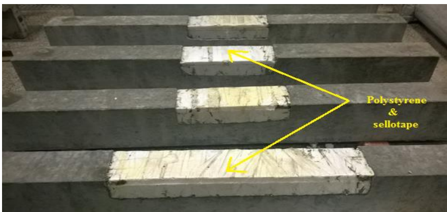
Figure 3.11. Polystyrene material placed into the damaged area and fixed using a sellotape after demoulding of RC beams.
