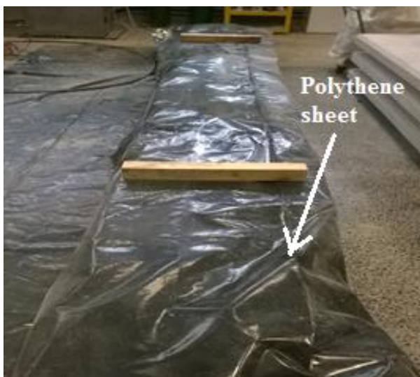
Figure 3.5. Curing of beams after demoulding.
