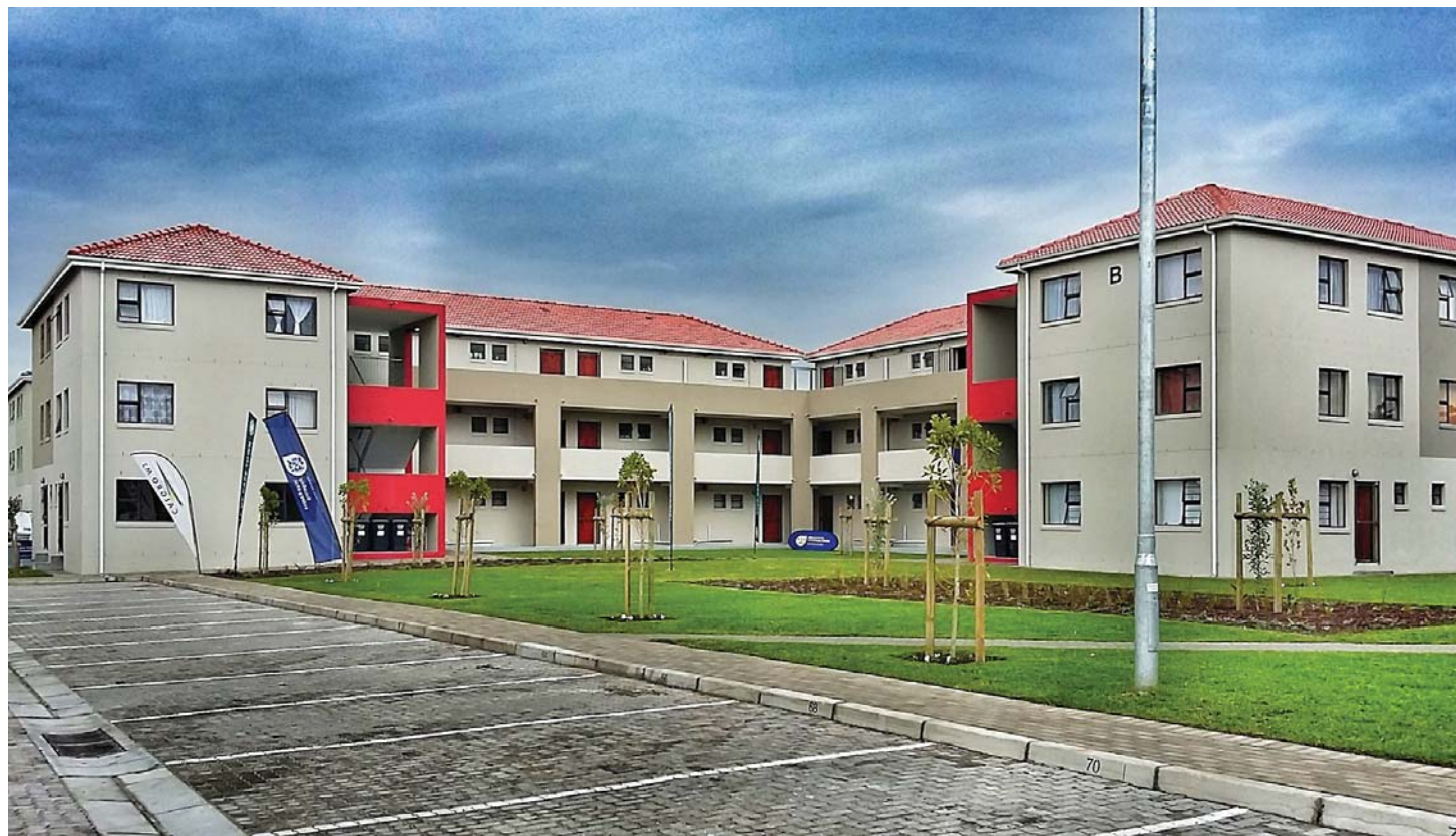
Figure 4.25 Belhar Affordable Housing Project (Source: http://www.calgrom3.com/index.php/belhar )
