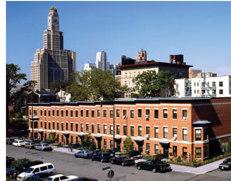
Figure 4.19 Townhouses in Brooklyn, New York (Source: http://moncon.com/projects/atlantic-center-phase-1-and-2/ )
