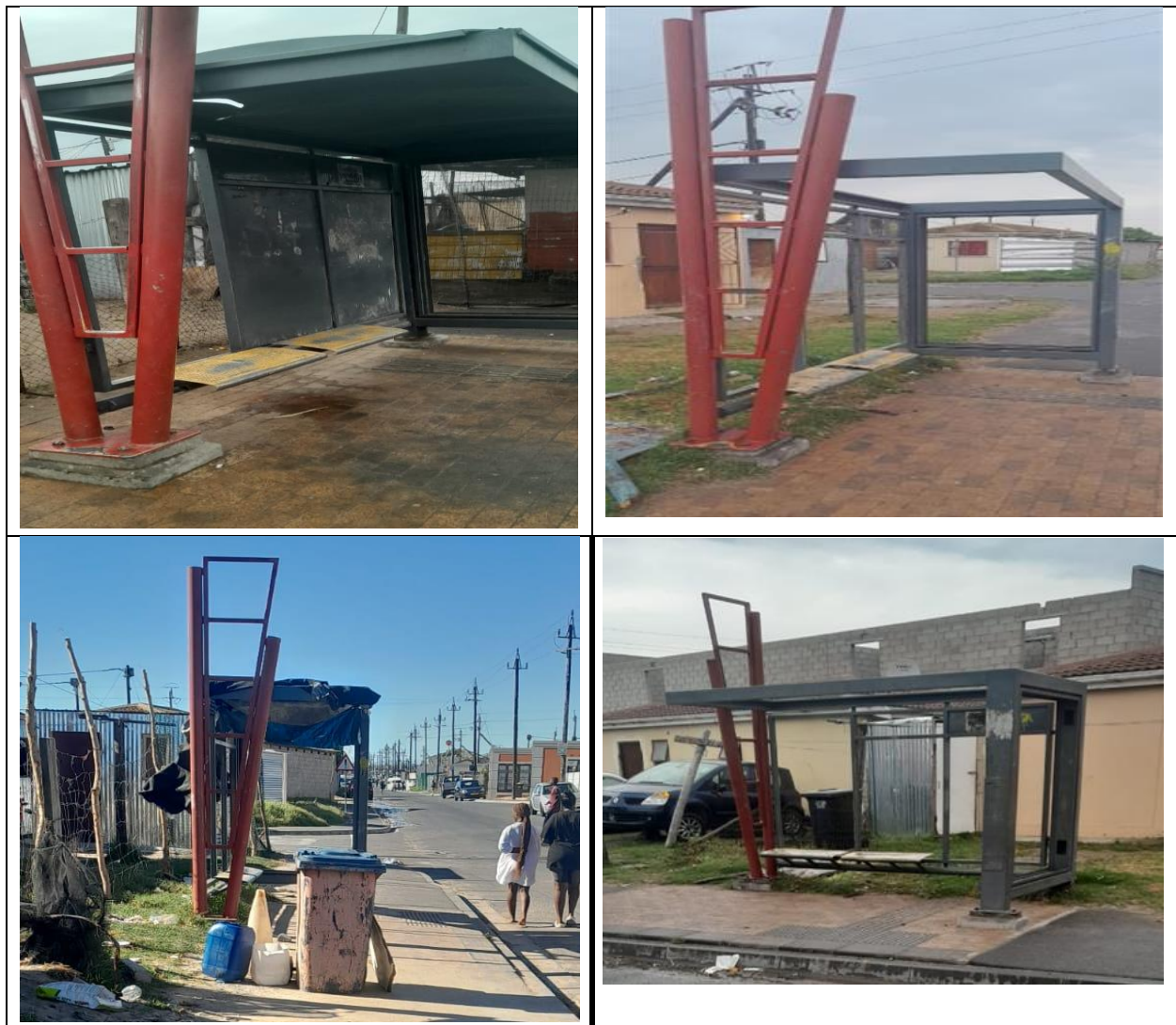
Figure 37: Idle MyCiTi bus stop infrastructure within Witsand
