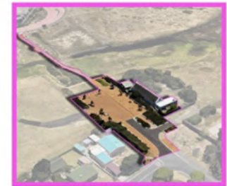
HERITAGE: KLEIN ZOAR PROVIDES HERITAGE SIGNIFICANCE TO WEMYSS STREET WHICH COULD BE A POTENTIAL MAJOR EAST WEST LINK ROAD
