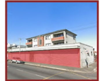
POOR URBAN IMAGE: WAREHOUSE/SHED BUILDING TYPOLOGY WITH BLANK FACADE DETRACT FORM ACTIVITY SPINE PRINCIPLES
