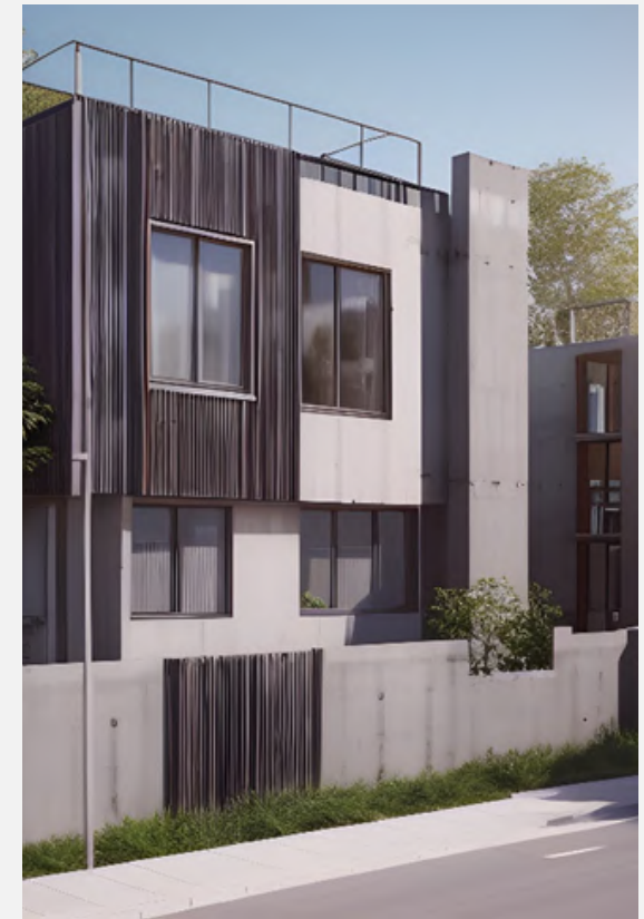
Figure 11 Render illustrating various elements that can enhance aesthetics of the building, different materials, textures, presence of trees, depth in the façade. By Author
