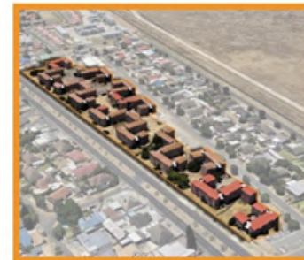
SOCIAL HOUSING: ALBOW GARDENS - A VERY SUCCESSFUL HOUSING PROJECT ON KOEBERG RD
