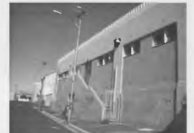
Necessary back entry: Clyde Street
