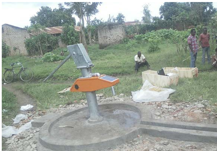
Figure 15: Solar powered smart borehole
