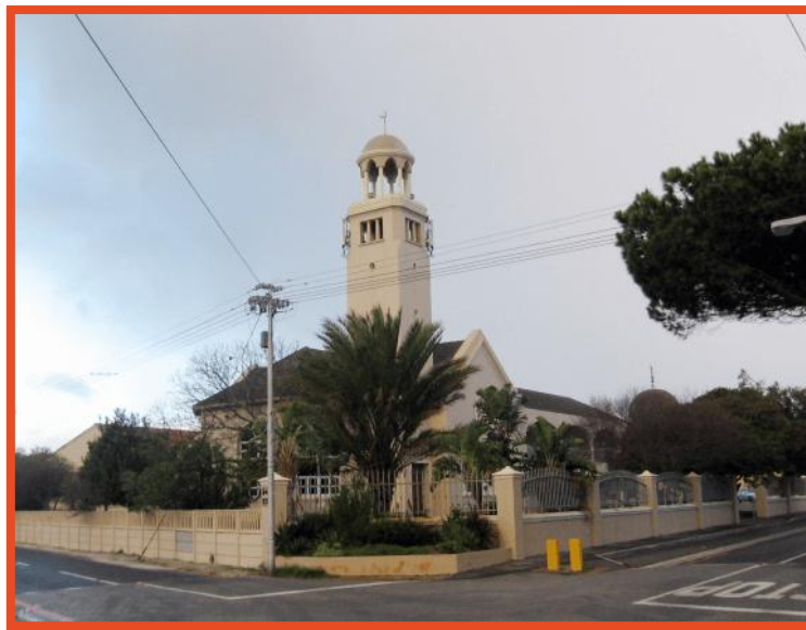
Figure 10: Image of mosque after downpour of rain
