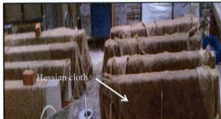
Figure 3.8: Beams being cured by covering with hessian cloth
