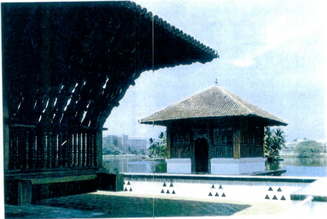
Plate 4.5- View to the end pavilion of the temple clearly showing the effect of deep eaves (Source: Taylor, B. B., 1995, pp. 162)
