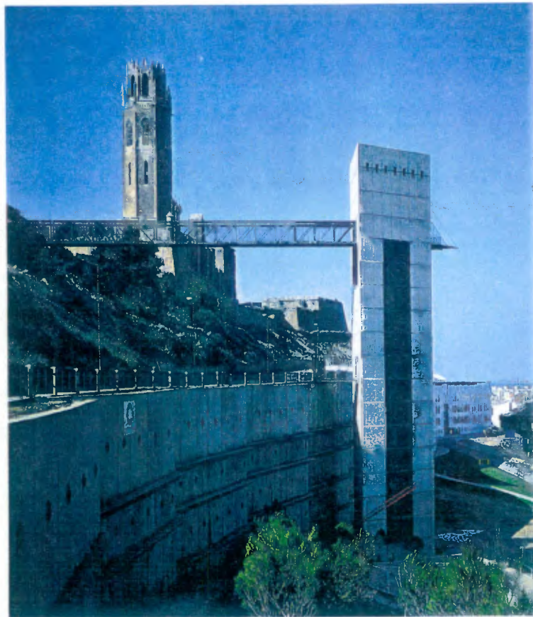
Plate 4.9- The Canyeret development showing the elevator tower and bridge. (Source: Tzonis, A. and Lefaivre, L., 1992, pp. 238)
