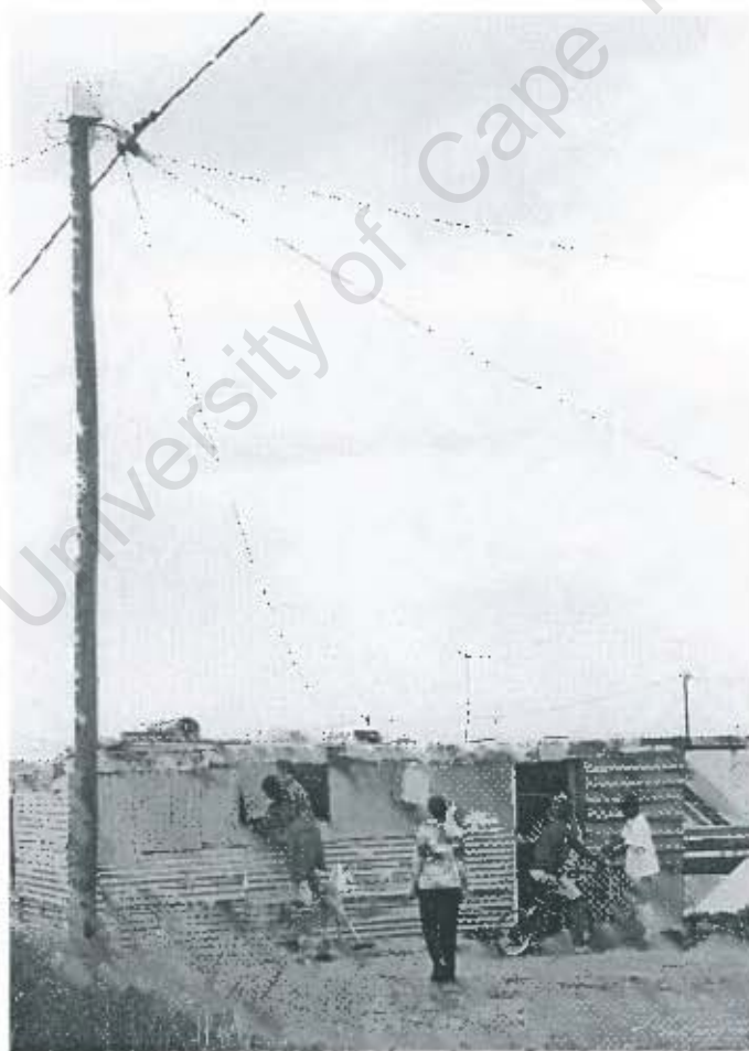
Figure 4-8: Orange Farm in 1999 - wooden poles and external meter boxes.
