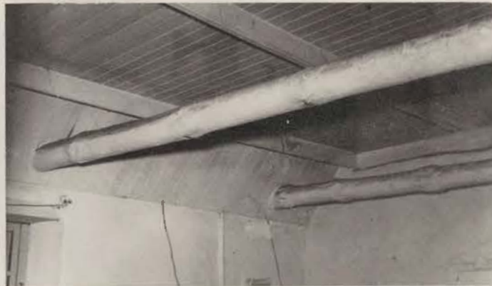
12. Silver Tree poles in the roof construction of early buildings in Wynberg. These survive in the long structure which was certainly the Military Hospital, and may also have been at one time the Military Chapel.
