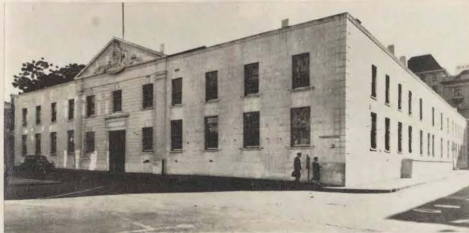
Old Supreme Court Building.
