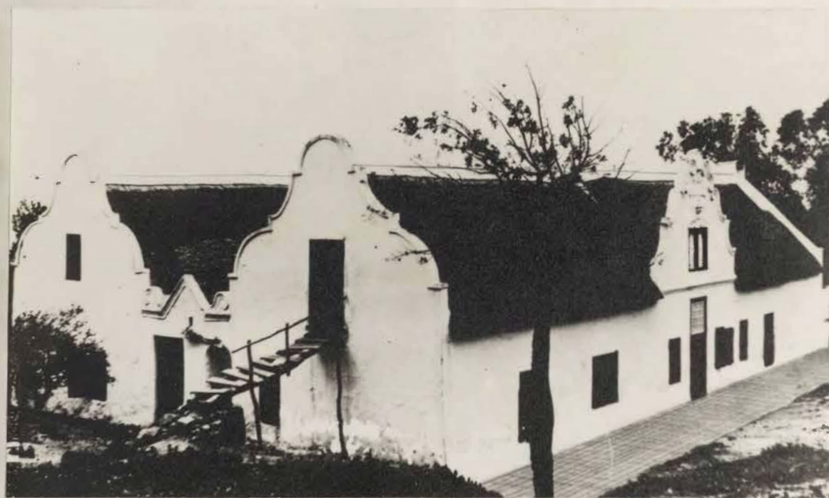
11. Typical Cape eighteenth Century farmhouse: 'Paarl Diamant' with an H plan, Baroque side gables and Rococo centre gable. (The photograph has been retouched to remove flood damage. Elliott.)
