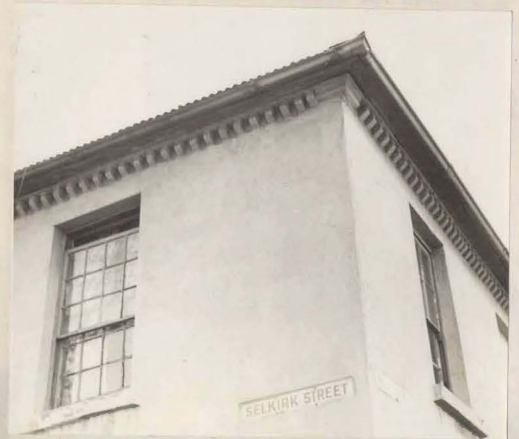
56. Brick house with brick corbel eaves. New Market area, Cape Town.
