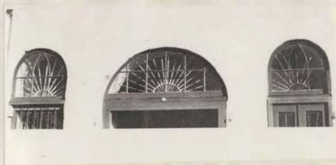
69. Detail of the warehouse in Plate 71, showing the burglar guards inside the ground storey fanlights.
