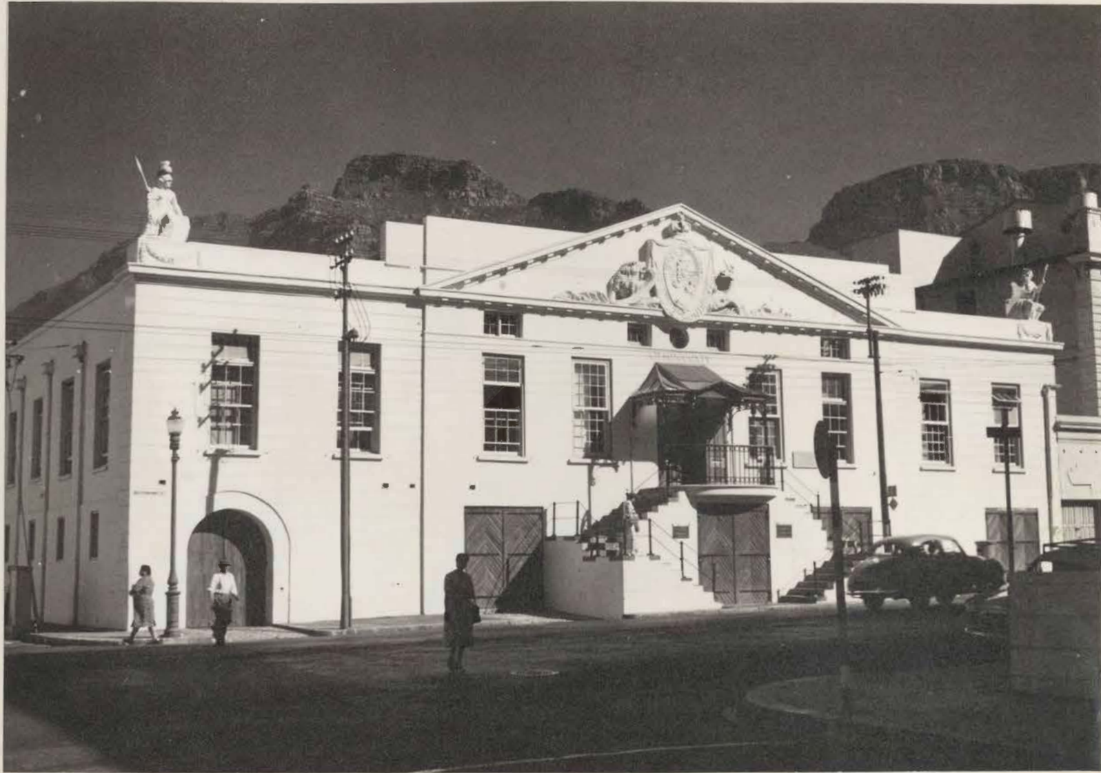
23,24. The Customs House of 1814. (The canopy over the doorway was added c.1880. The windows flanking it are original, but not the clerestory windows under the pediment).
