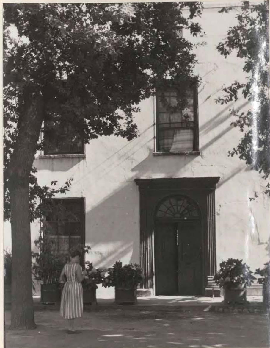
26. House in Dorp Street, Stellenbosch. The frames in this case are recessed behind wooden reveal linings, a common Georgian detail. Originally the wall was probably a medium or dark tone, the window joinery, reveal linings and door surround light.
