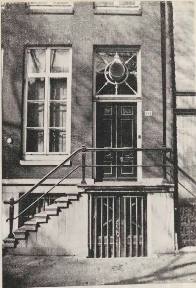
2. Doorway and Fanlight in Amsterdam. ± 1800.
