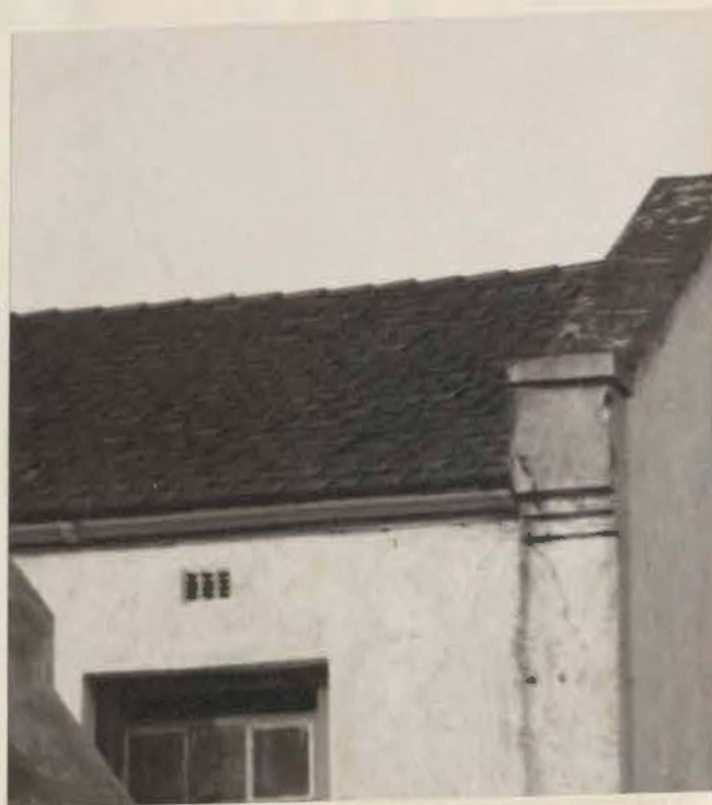
55. Shingle roof in District Six, Cape Town.
