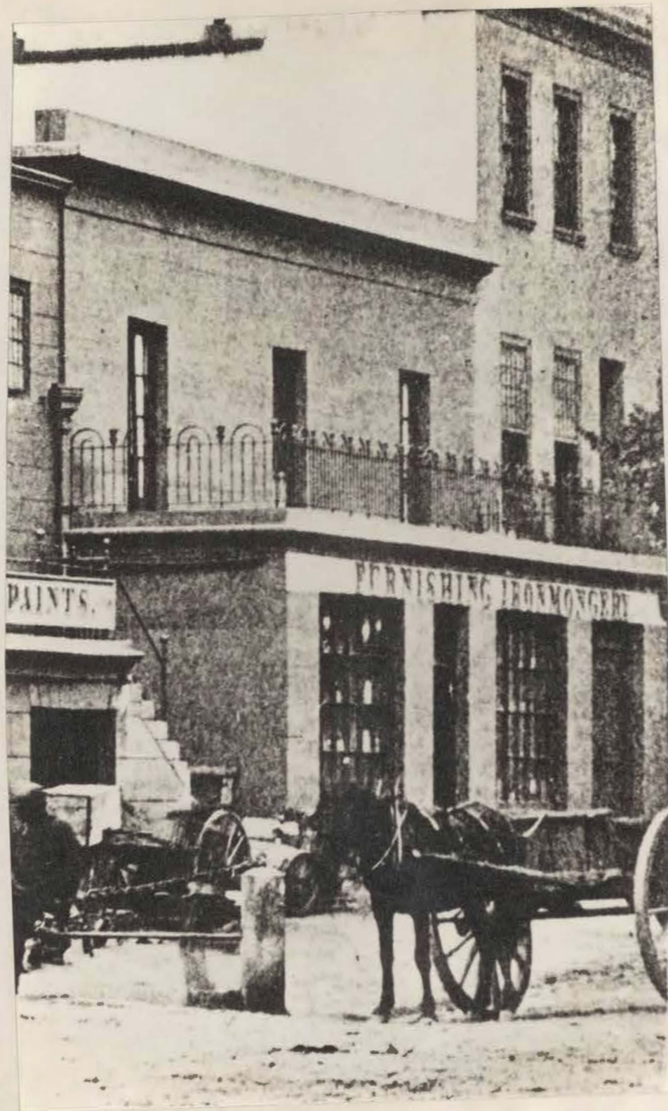
79, 80. Railings in Strand and St. George's Streets, Cape Town. The building at the right, with its balconies, steep railings and circular headed fanlight, is a typical Cape Regency house.
