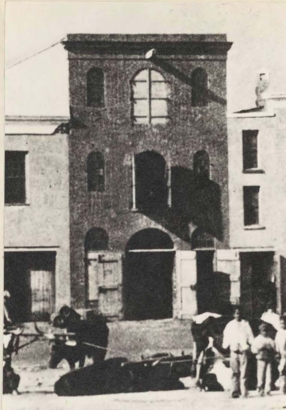
71. Brick warehouse in Riebeeck Square, 105, Bree Street (cf. Plate 73). (Africana Museum).
