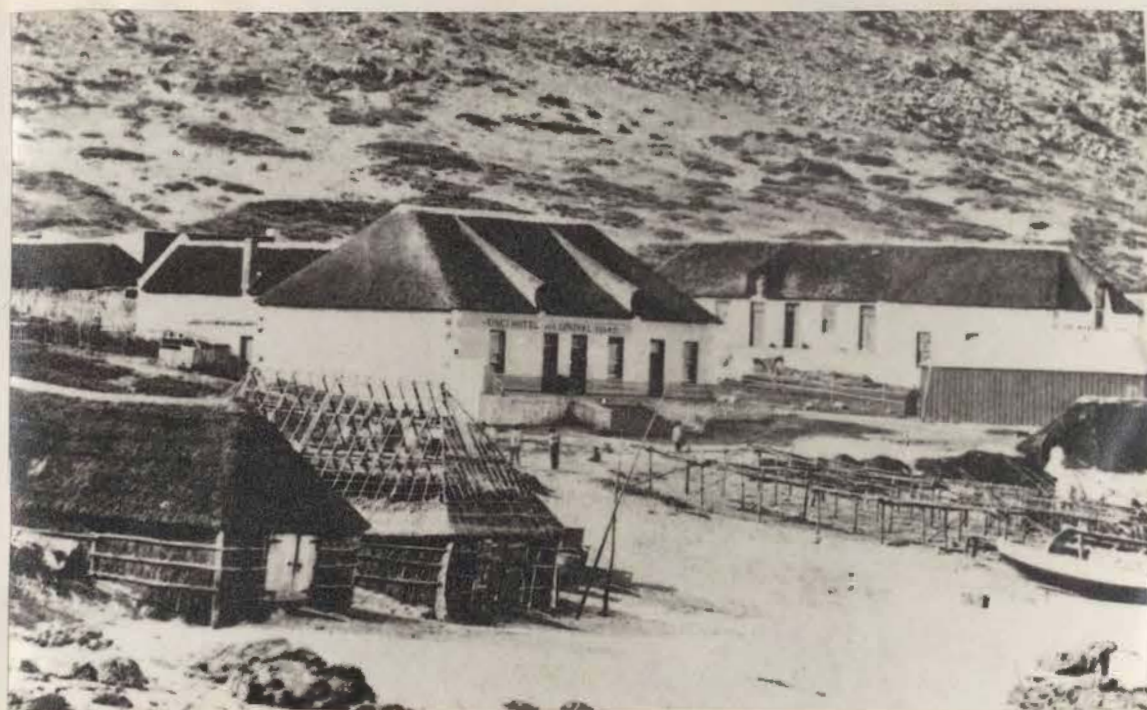
6. The buildings thought to be those of Kalk Bay Fisheries, an early photograph. (Note the timber framed and wattled huts in the foreground, of the same type as the Wynberg military quarters).
