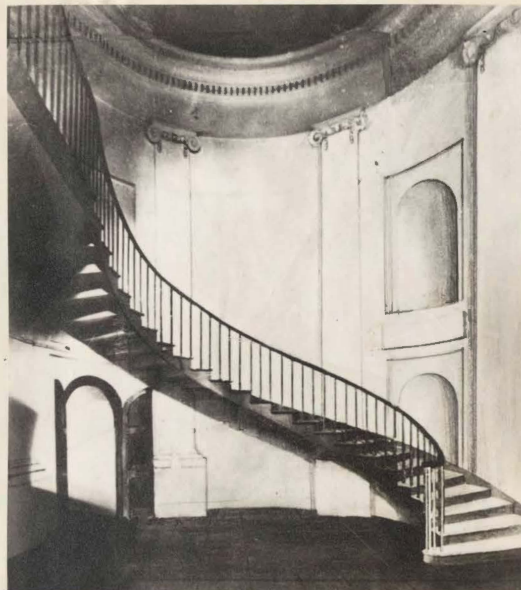
11. One of the twin staircases of the old Supreme Court vestibule. (A composite restoration of its original appearance from a number of photographs taken by Arthur Elliott & Jeffrey during its demolition).
