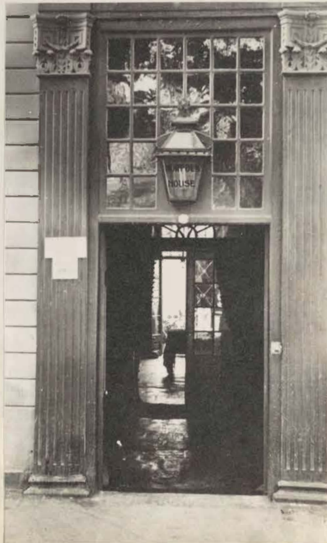
34. 'Norfolk House', Strand Street, Cape Town, dated 1799. Entrance doorway and hall. (Elliott).
