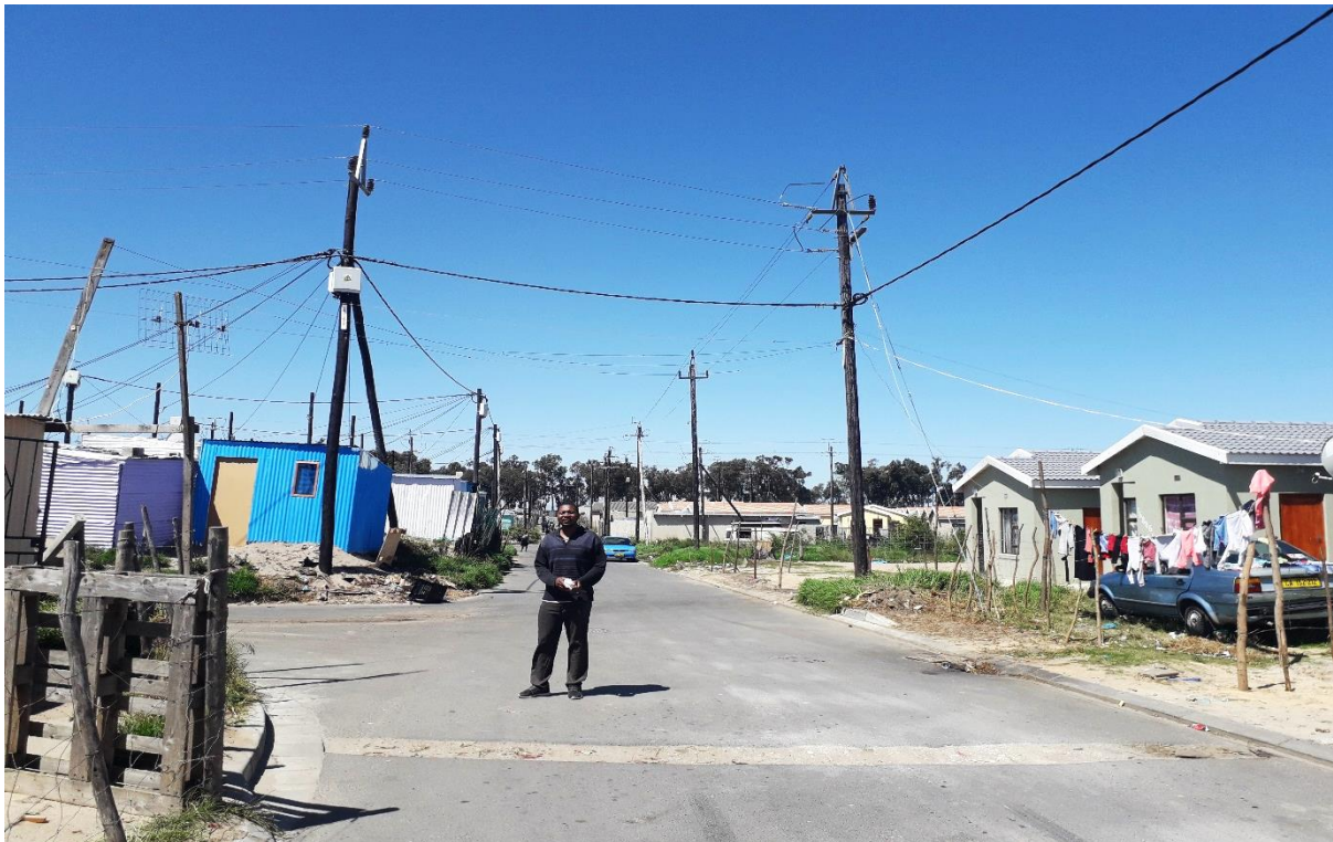
Figure 4: Non electrified RDP houses tapping electricity from Eskom poles.
