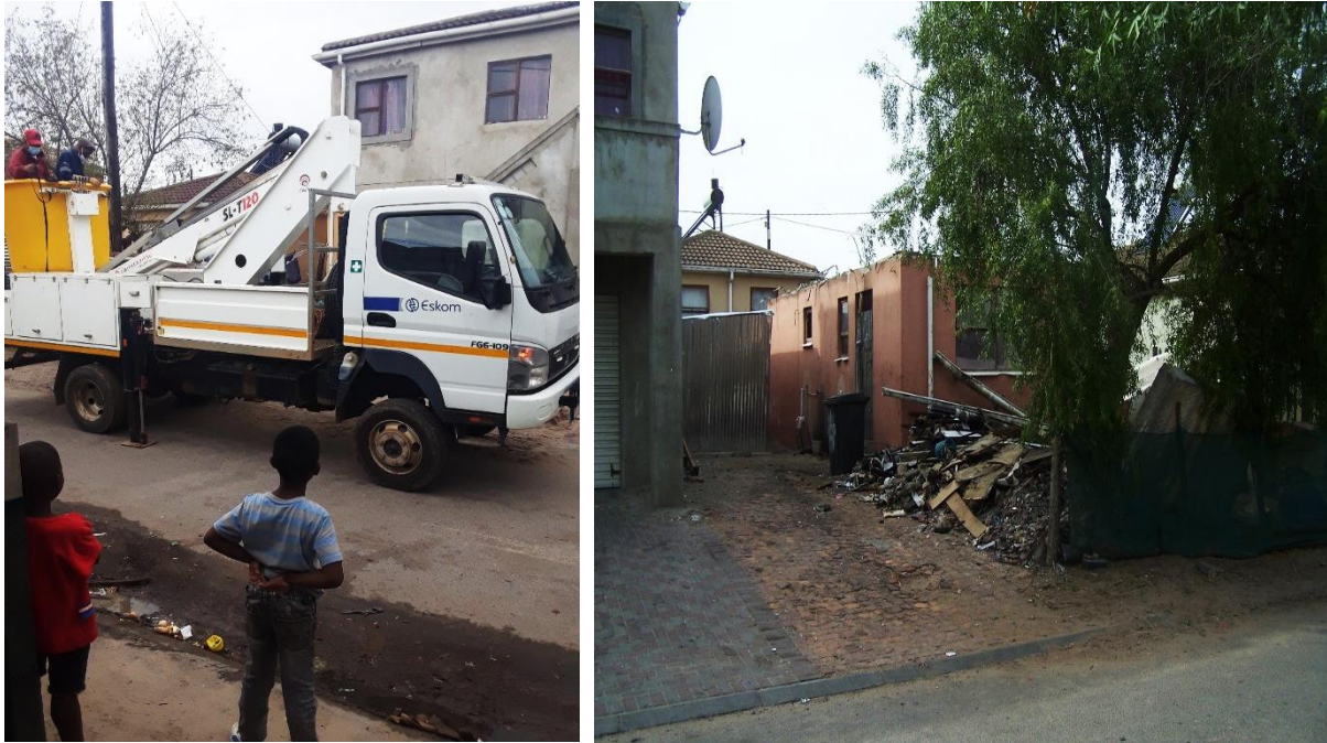
Figure 13: RDP house gutted down in resident-made electricity connections related fire. The image on the left shows Eskom personnel who were called to avert the electricity fault, to the right is the RDP house burnt down in the fire (Source: Author, March 2021).
