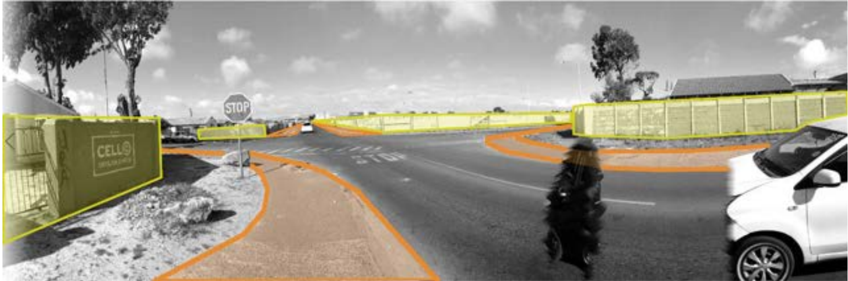
EXISTING STREET CONDITIONS
