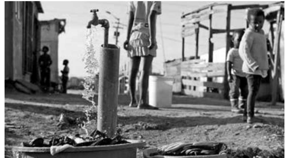
FIG 1.6: Failing water and sanitation infrastructure (African centre for Green Economy,2016)
