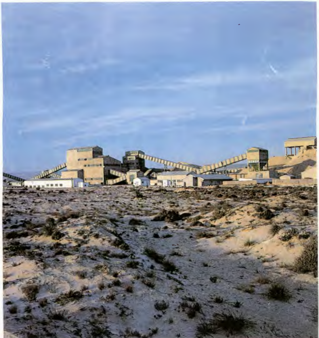
TREATMENT PLANT - KLEINZEE
