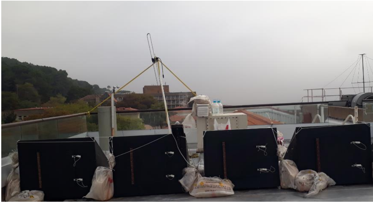
Figure 3.10: Layout of equipment on the roof – Back Side.
