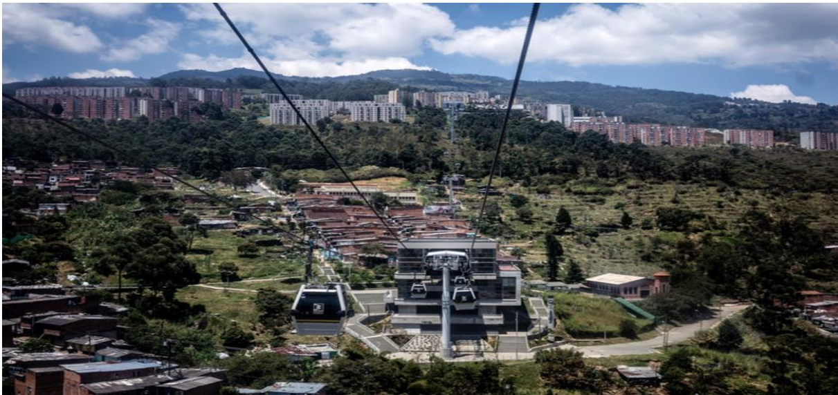
Figure 3.7: Image depicting the Metrocable in Medellín (Milton, 2017).
