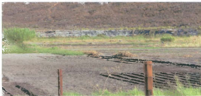
Figure 5.12: Upper package of primary exposure visible from behind the levee on the opposite bank
